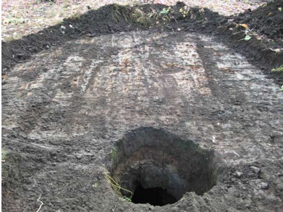
Fig. 3 Collapsed mine shaft in foreground with plough scarred natural clay in the rear, from the north
