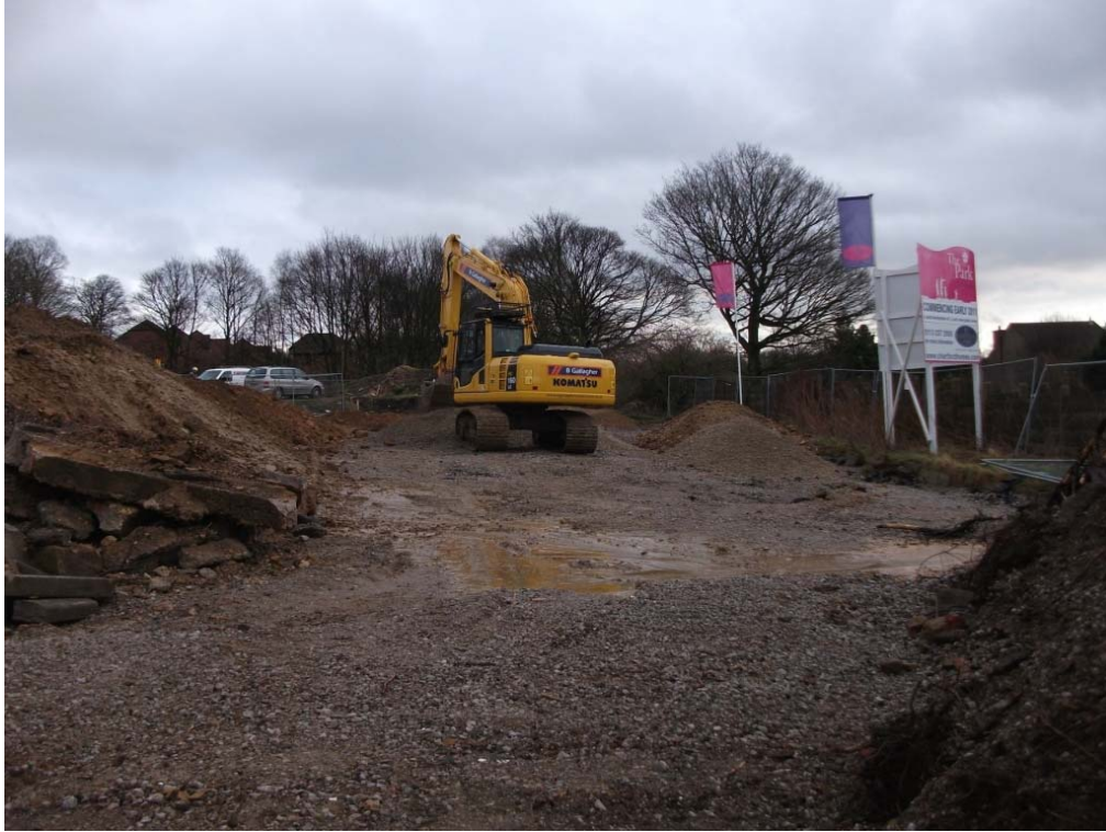
Plate 1: Trench 1: Pre-excavation, Looking East
