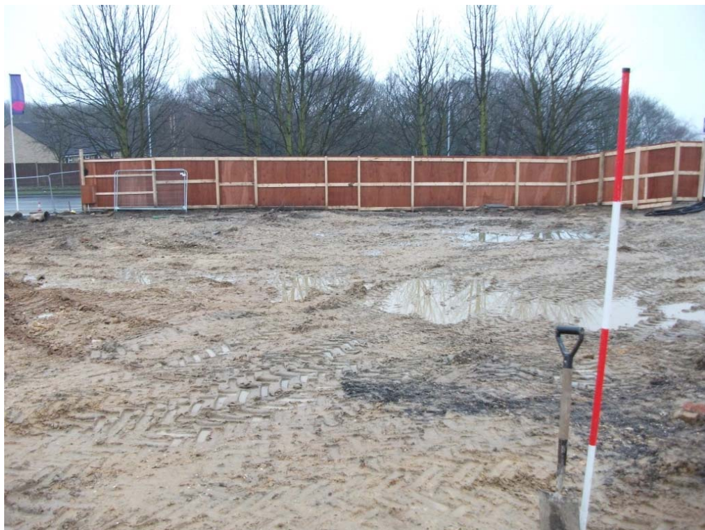
Plate 4: Trench 3, Pre-excavation, Looking Southwest
