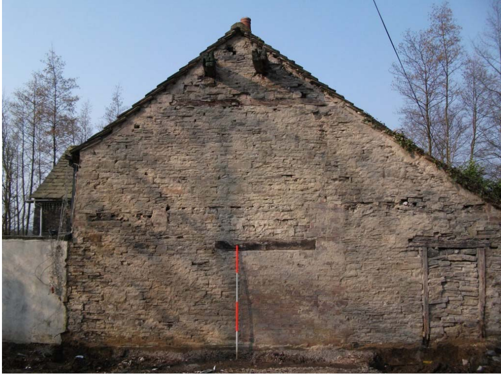
Plate 1: East-Facing Gable End of Cinder Hill Farm
