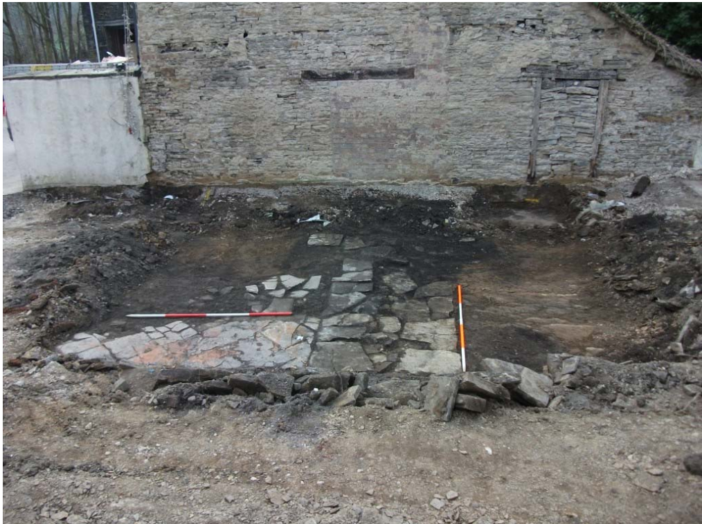
Plate 2: After Stripping, Pre-excavation, Looking North
