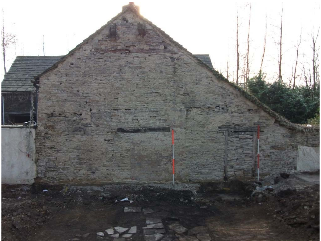
Plate 5: East Facing Gable End of Cinder Hill Farm
