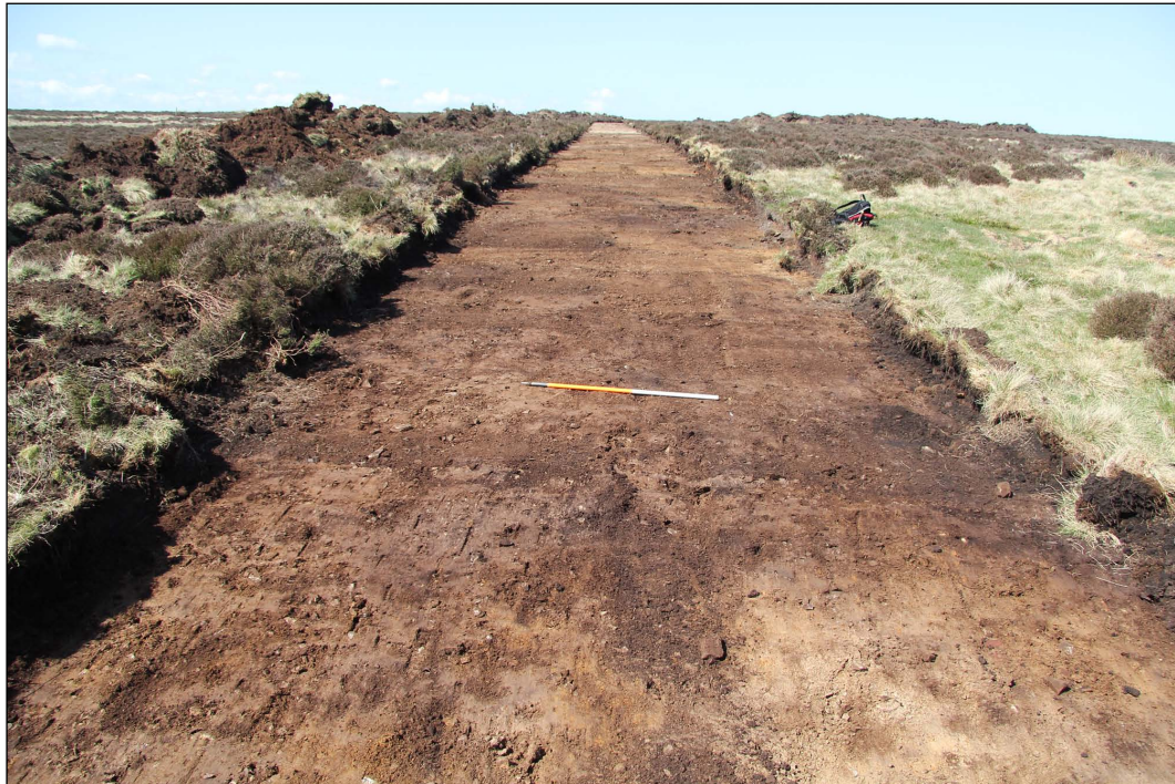
Fig 6 - Access track to WTG18
