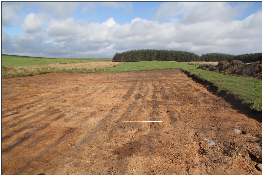
Fig 5 - General view of stripped area at WTG1, showing plough scores
