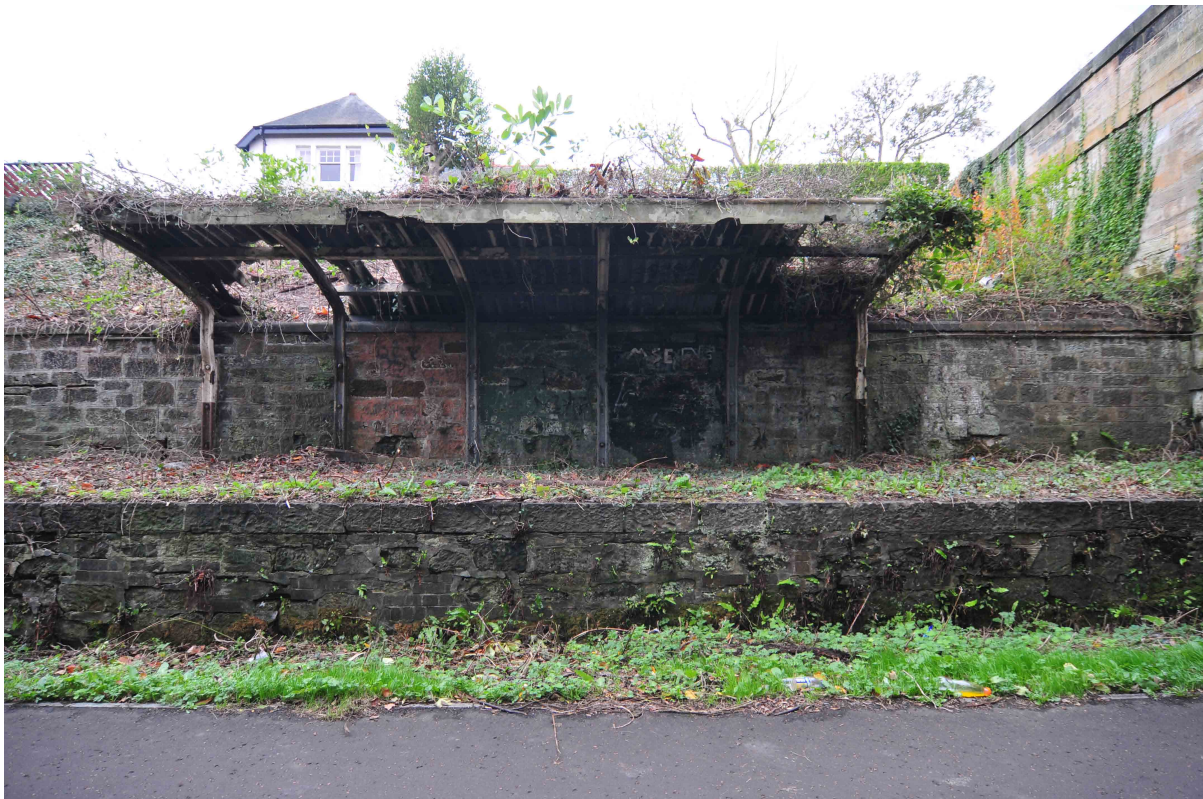
Plate 7 - Platform shelter situated on the west platform
