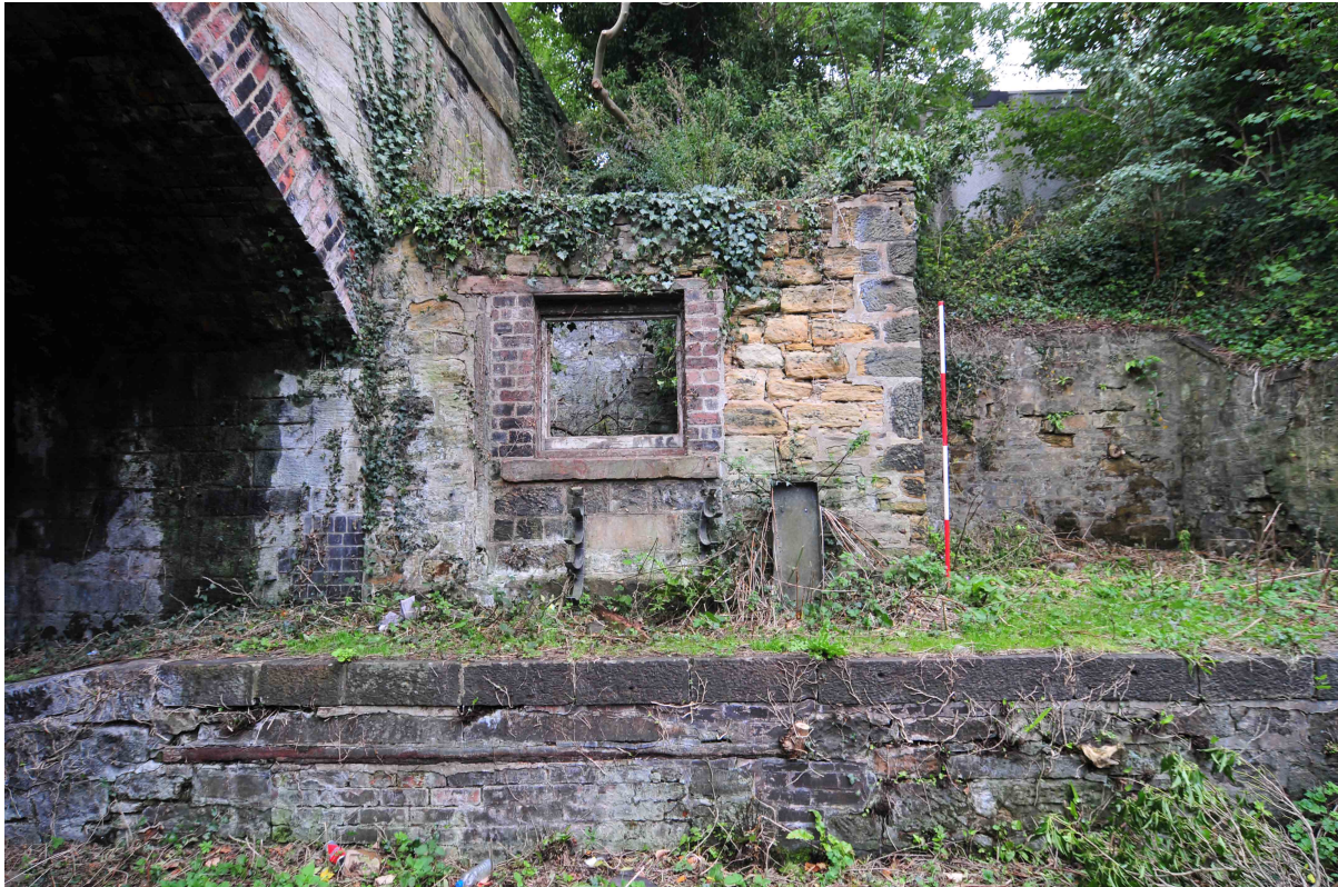
Plate 5 - West-facing elevation of Building 1
