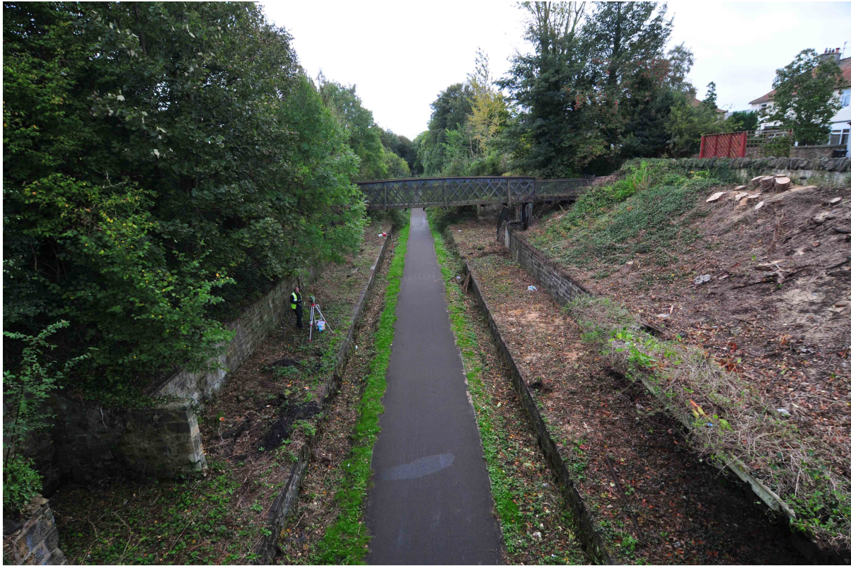
Plate 4 - General view of Eskbank Station looking south from the Lasswade Road Bridge
