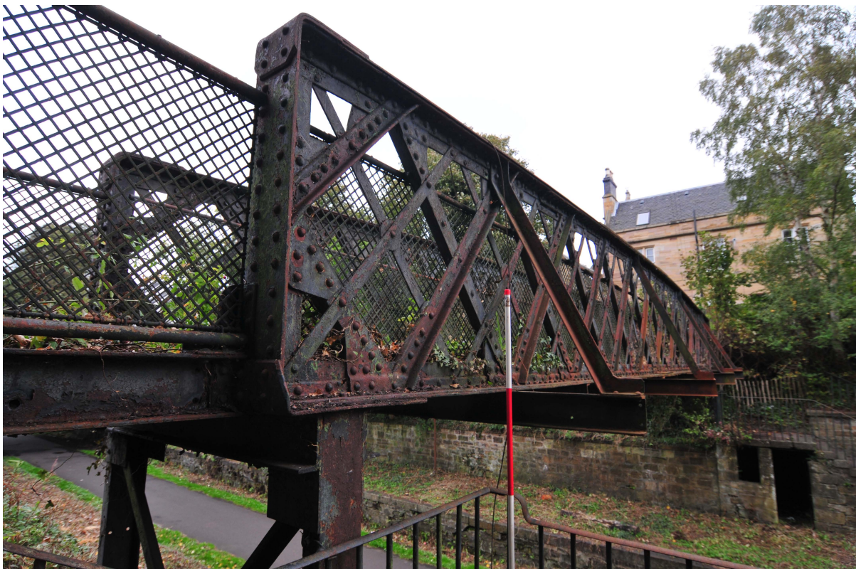
Plate 9 - Structural lattice work of the iron plate footbridge
