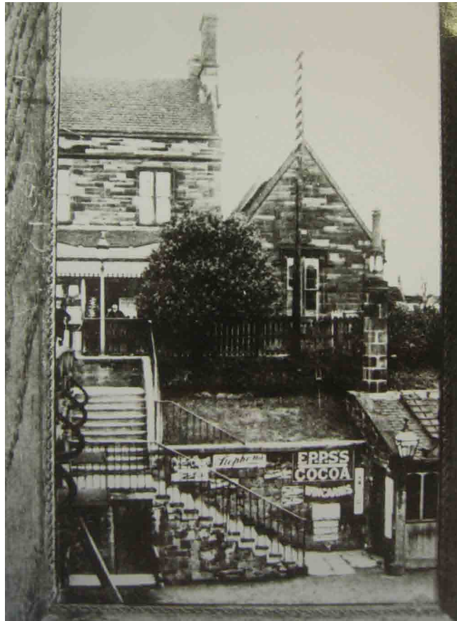
Plate 1 - A late 19th century photograph of part of the east platform and footbridge steps
