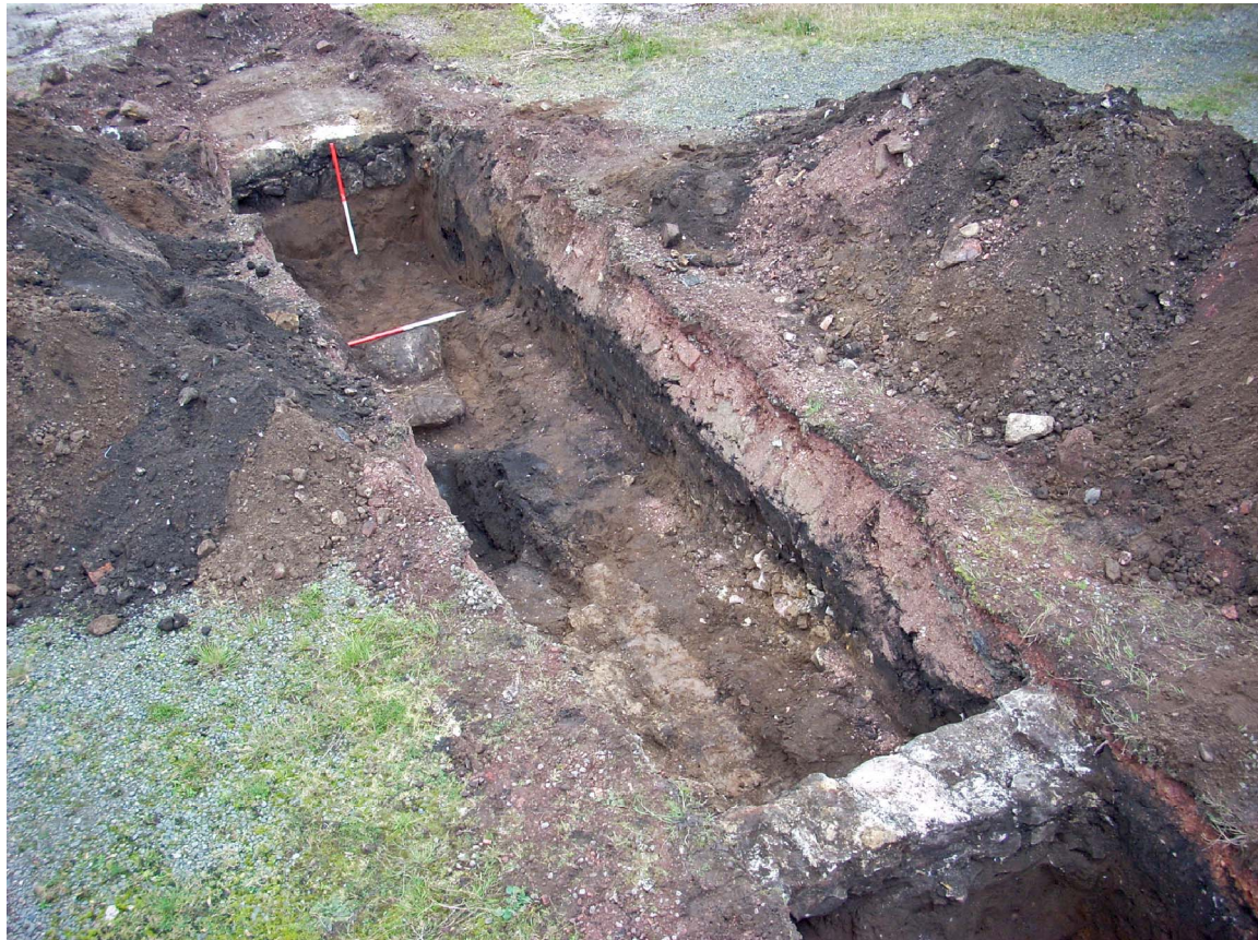
Fig 4 - The eastern end of Trench 1 from the WNW
