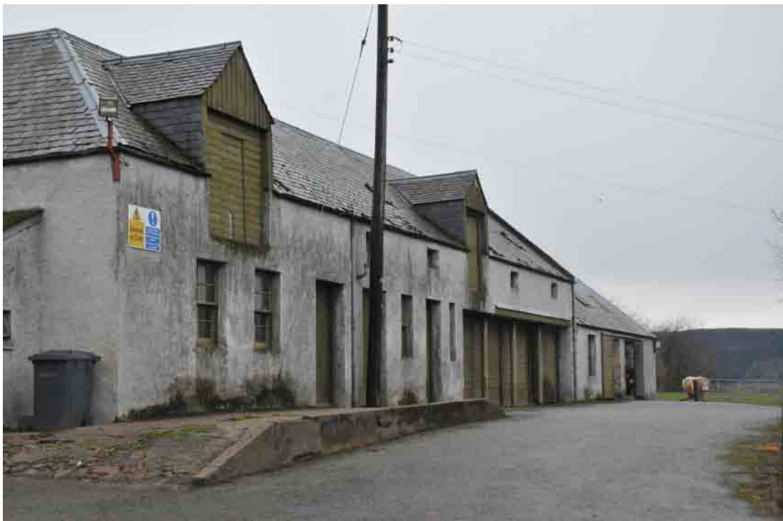
Fig 10 - West range from the north-east
