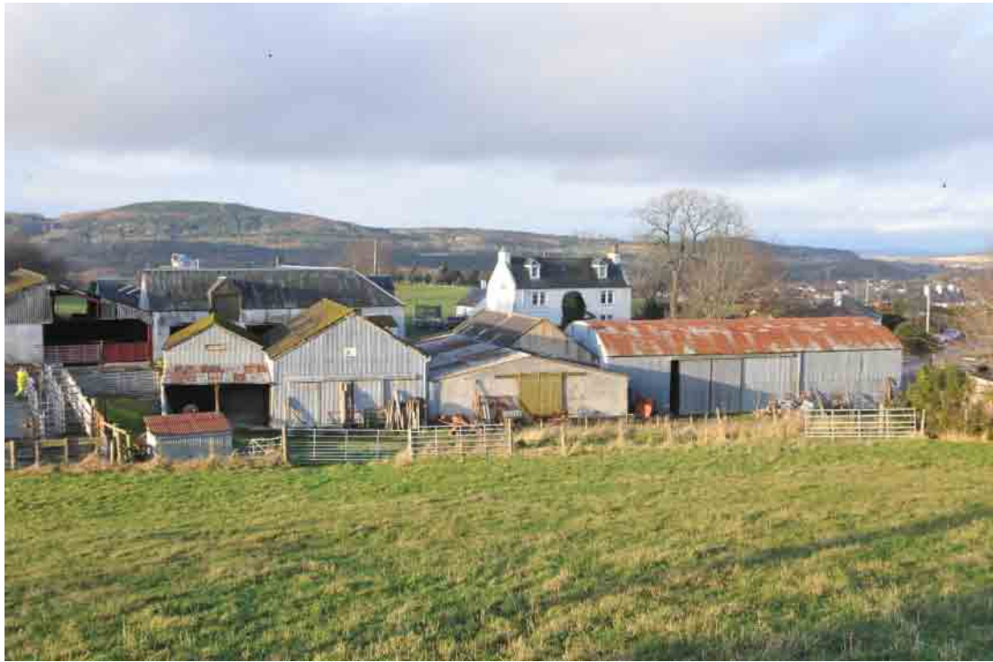
Fig 13 - General view of the farmstead from the south-east
