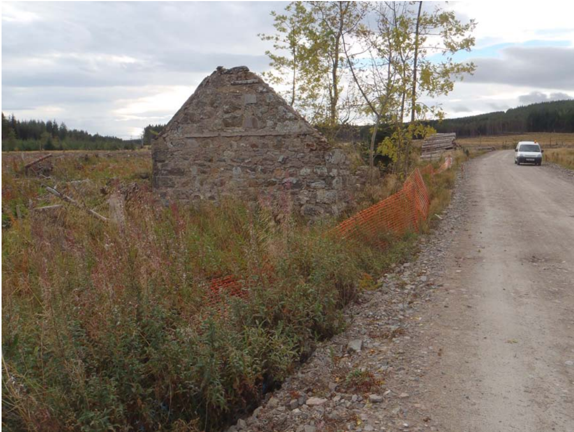
Fig 4 - Rosarie Farmstead post-construction, from north
