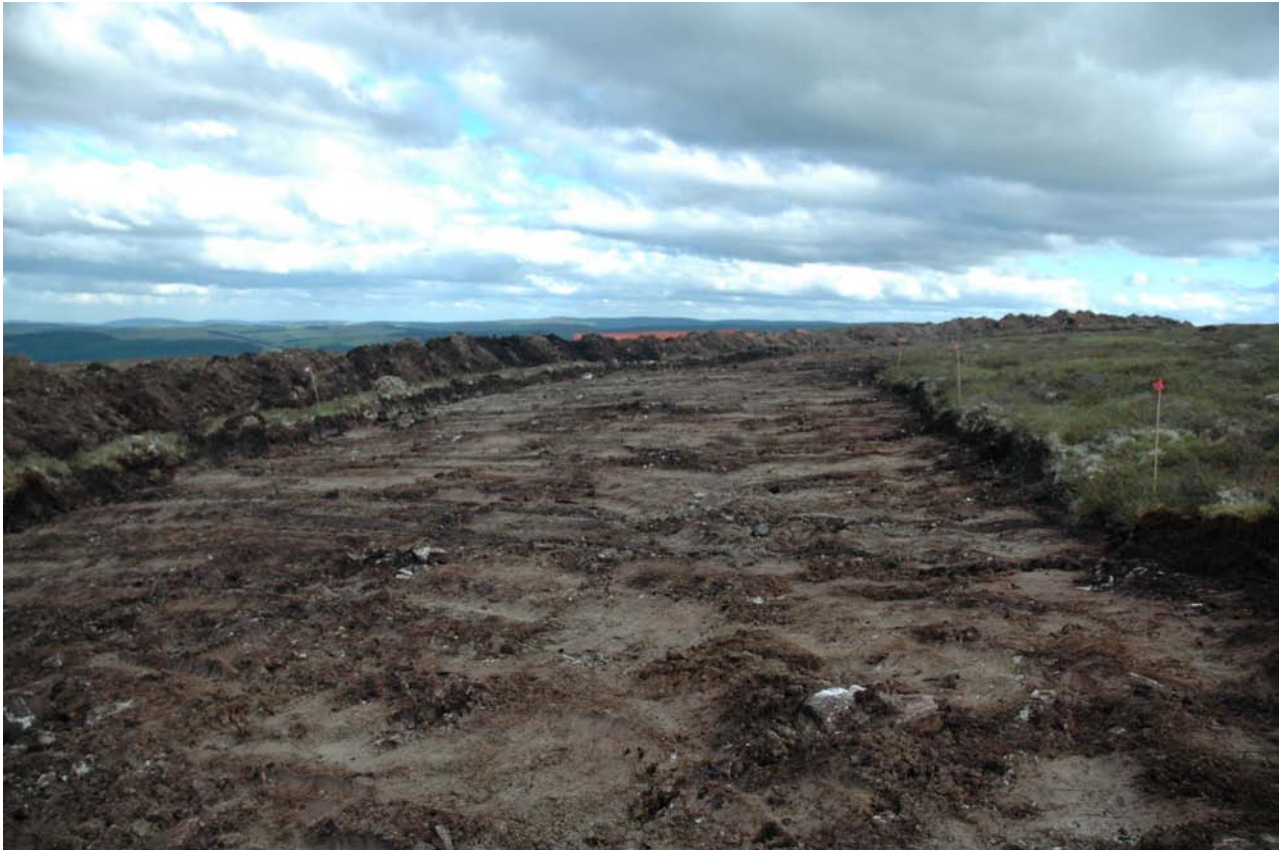
Fig 2 - General view of stripped area near T12, from north
