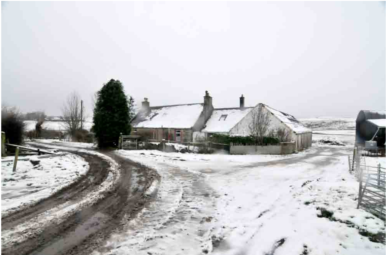
Fig. 21 General view of Riggfoot from south-east
