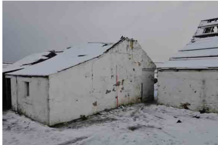
Fig. 15 North range, exterior from the south-west
