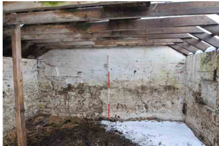
Fig. 16 North range interior. Unit 1 south-facing elevation
