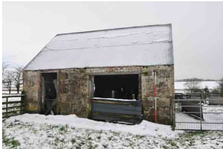
Fig. 19 Box barn exterior east-facing elevation
