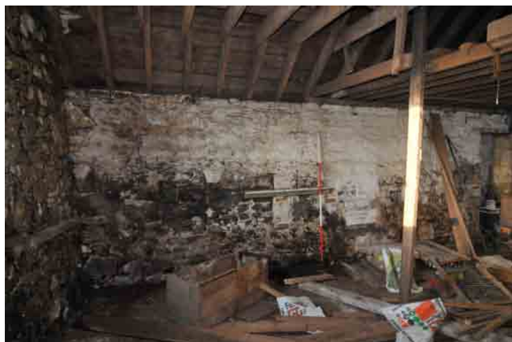
Fig. 11 West range interior, Unit 1 east-facing elevation
