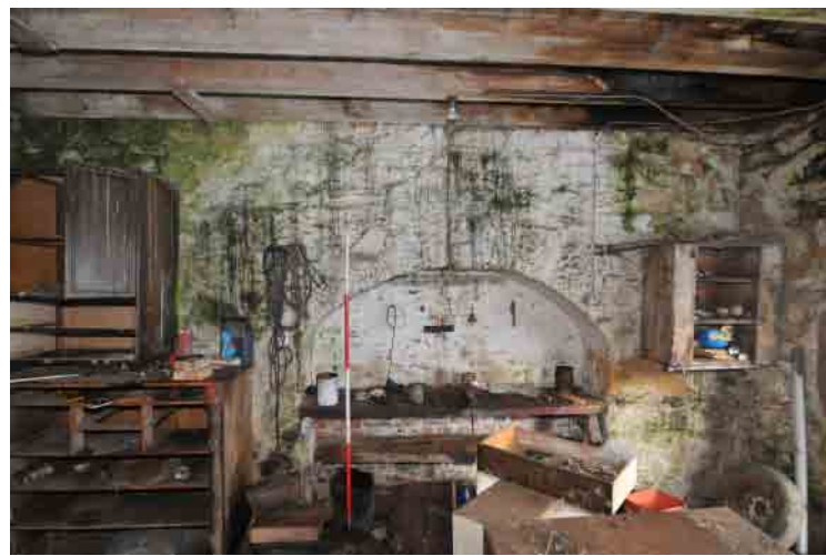
Fig. 13 West range interior. Unit 3 south-facing elevation
