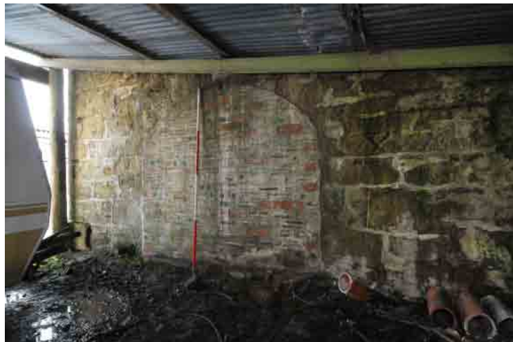
Fig. 10 West range exterior arch detail on north-facing elevation
