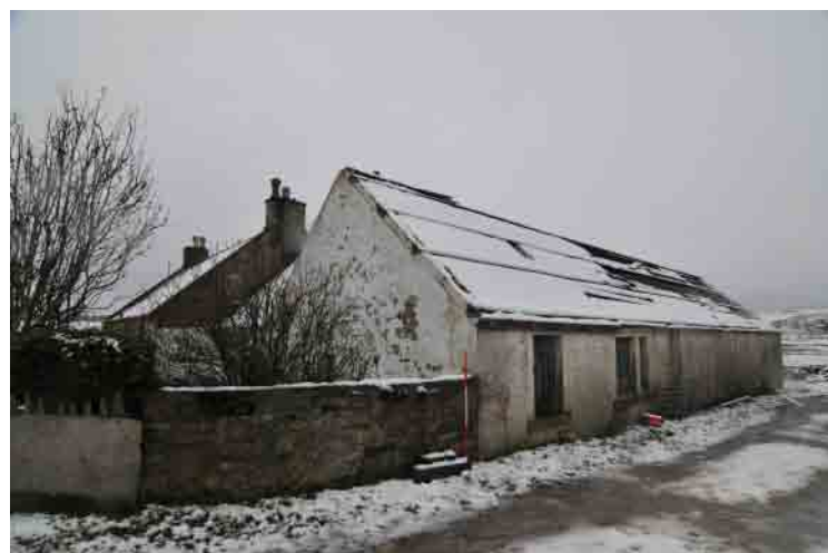
Fig. 17 East range exterior from the south-east
