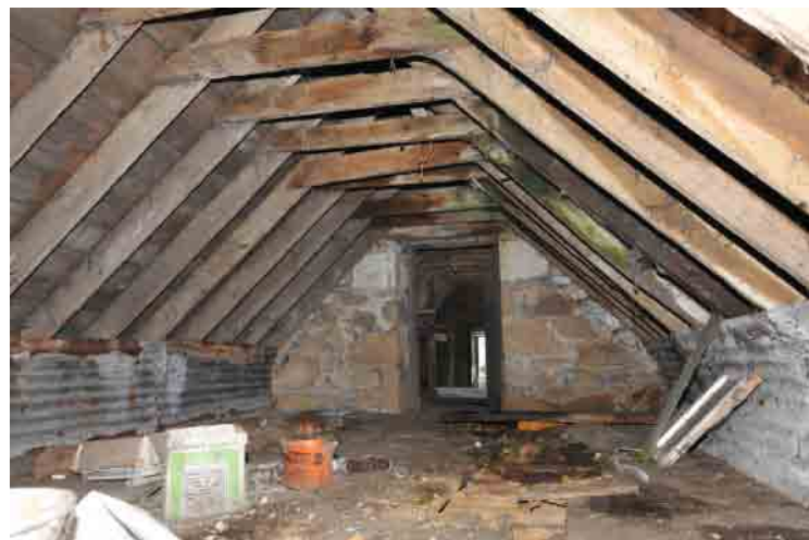
Fig. 14 West range loft from the south
