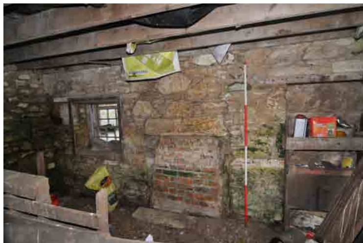
Fig. 20 Box barn interior south-facing elevation
