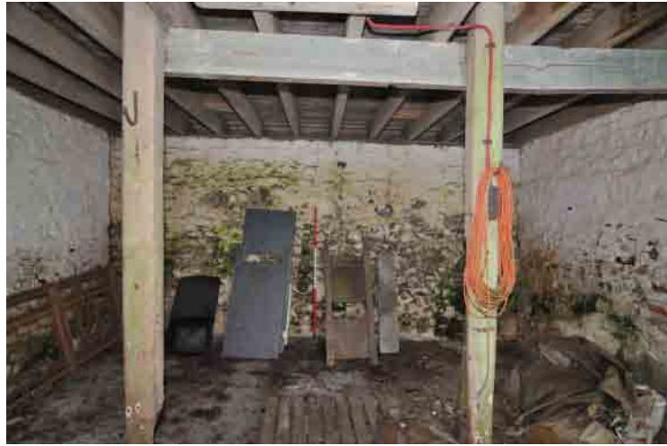
Fig. 12 West range interior, Unit 2, west-facing elevation
