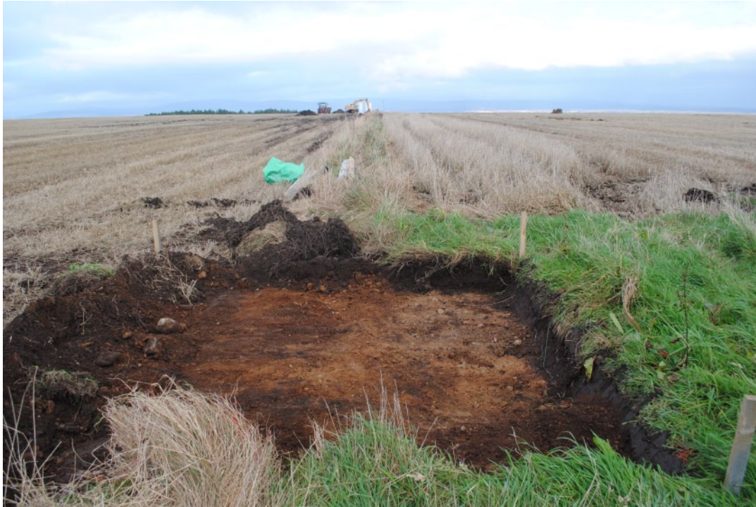
Fig. 2 Turbine control room site after clearance, from the south-east
