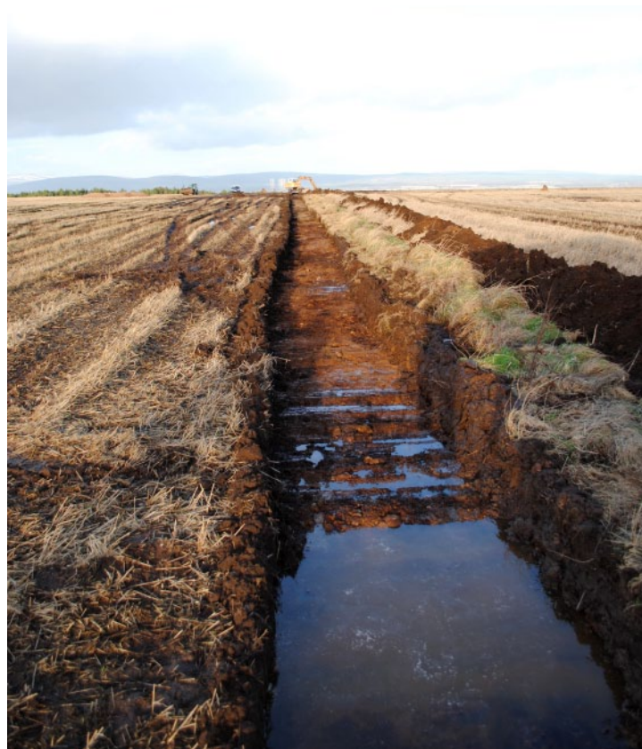
Fig. 5 Cable trench from south-east
