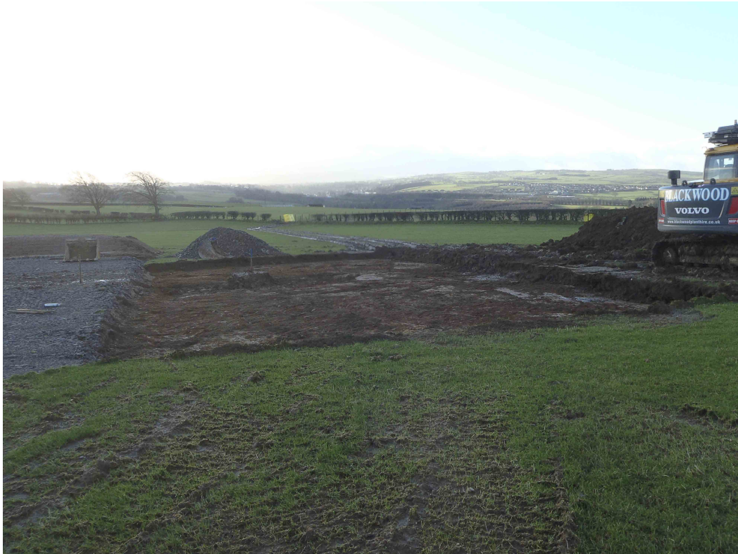
Fig. 2 - Turbine base stripped of topsoil
