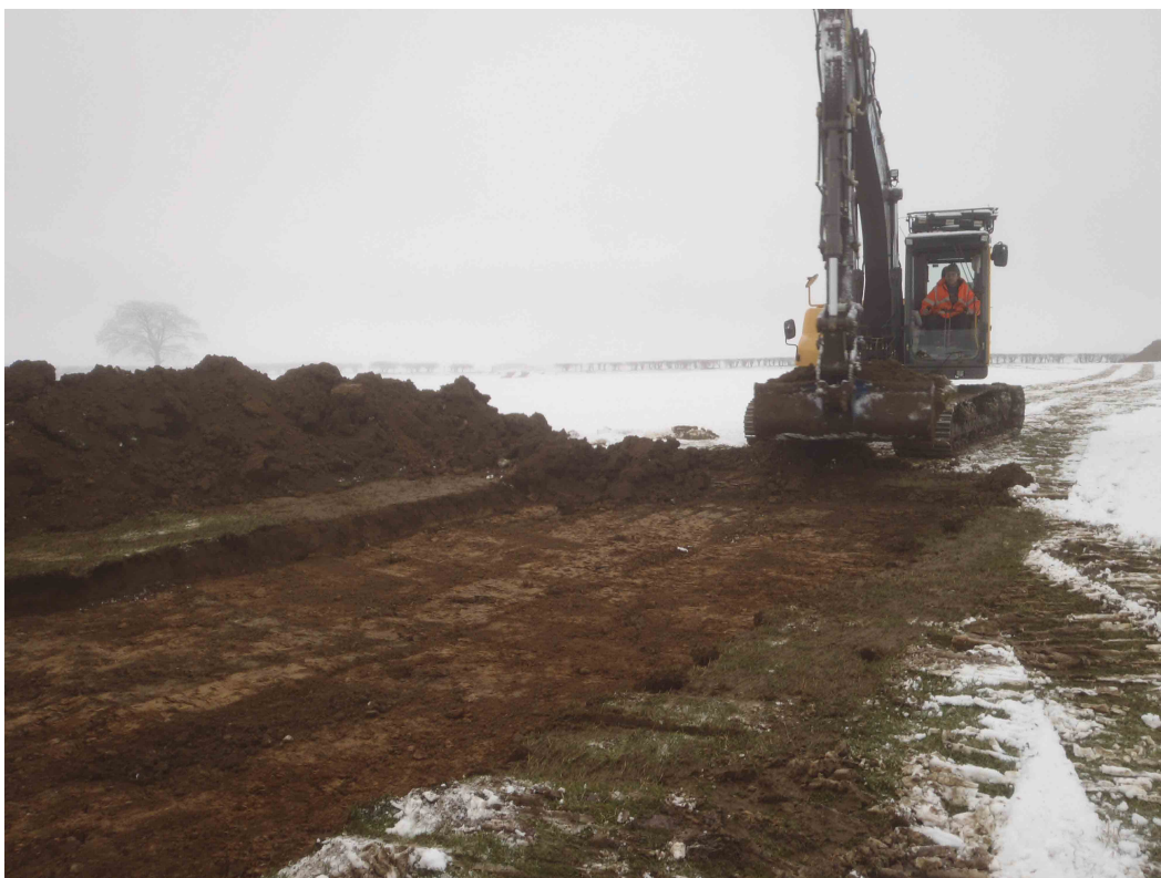
Fig. 3 - Topsoil stripping along access track
