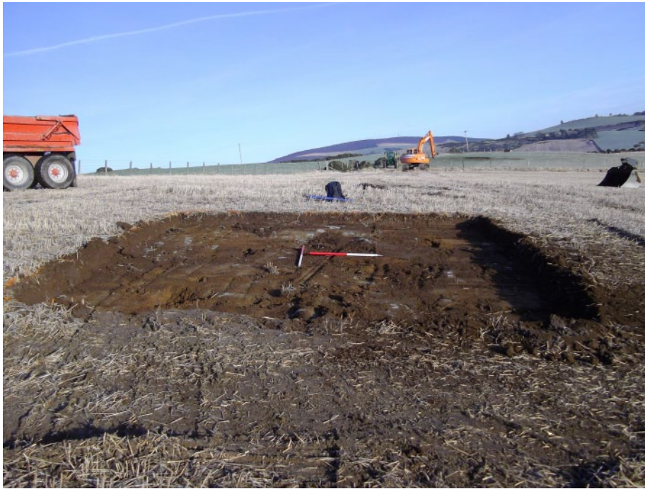
Fig. 2 The south-western turbine base from the south-west
