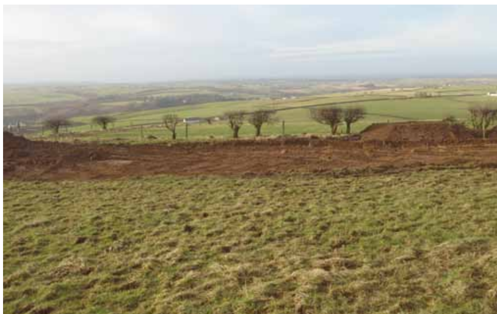
Fig. 4 - Turbine base 2 stripped of topsoil from east
