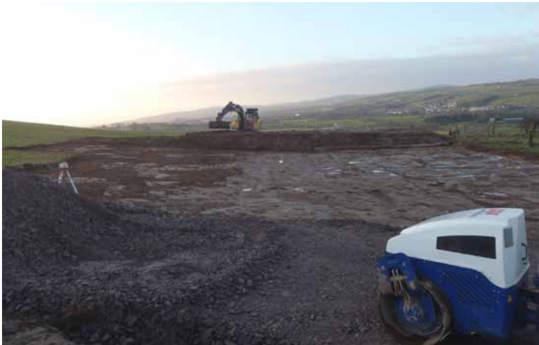
Fig. 3 - Crane pad stripped of topsoil from north-east
