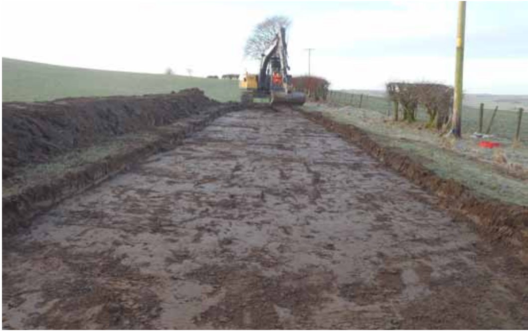
Fig. 2 - Topsoil stripping along access track
