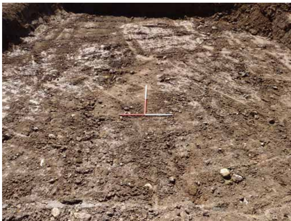
Fig. 5 - Turbine base 1 stripped of topsoil from north-east
