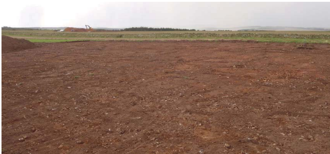
Fig. 4 - Stripped area around Wind Turbine 2, south west facing
