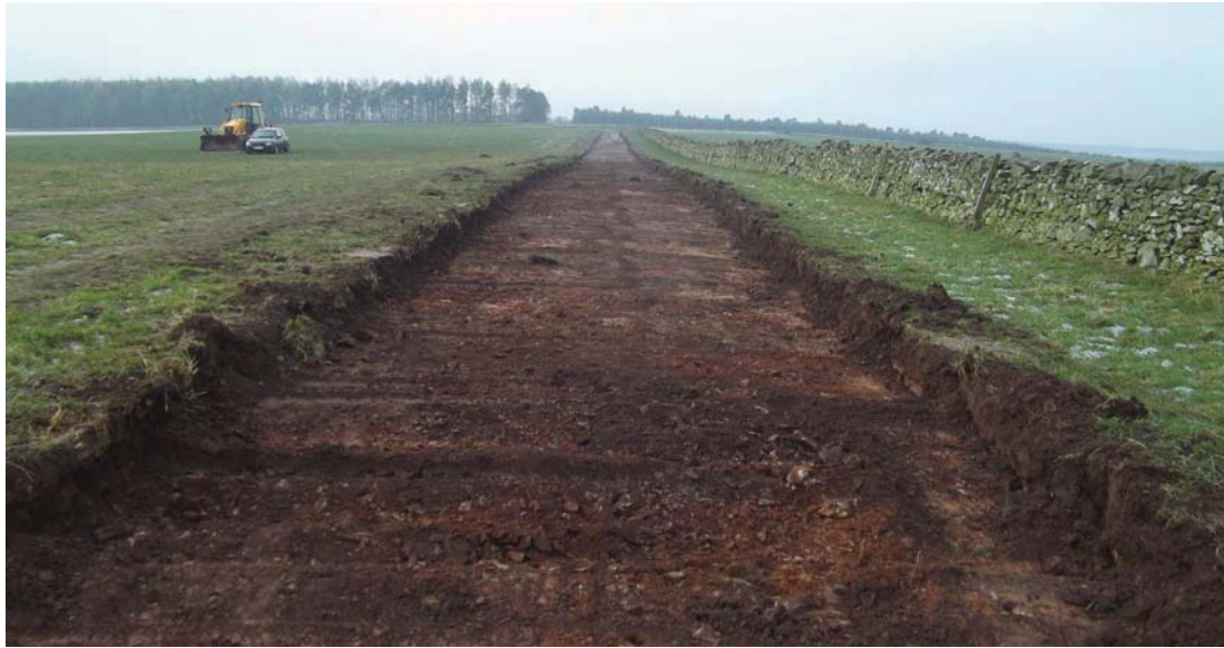
Fig. 2 - Access road facing southwest
