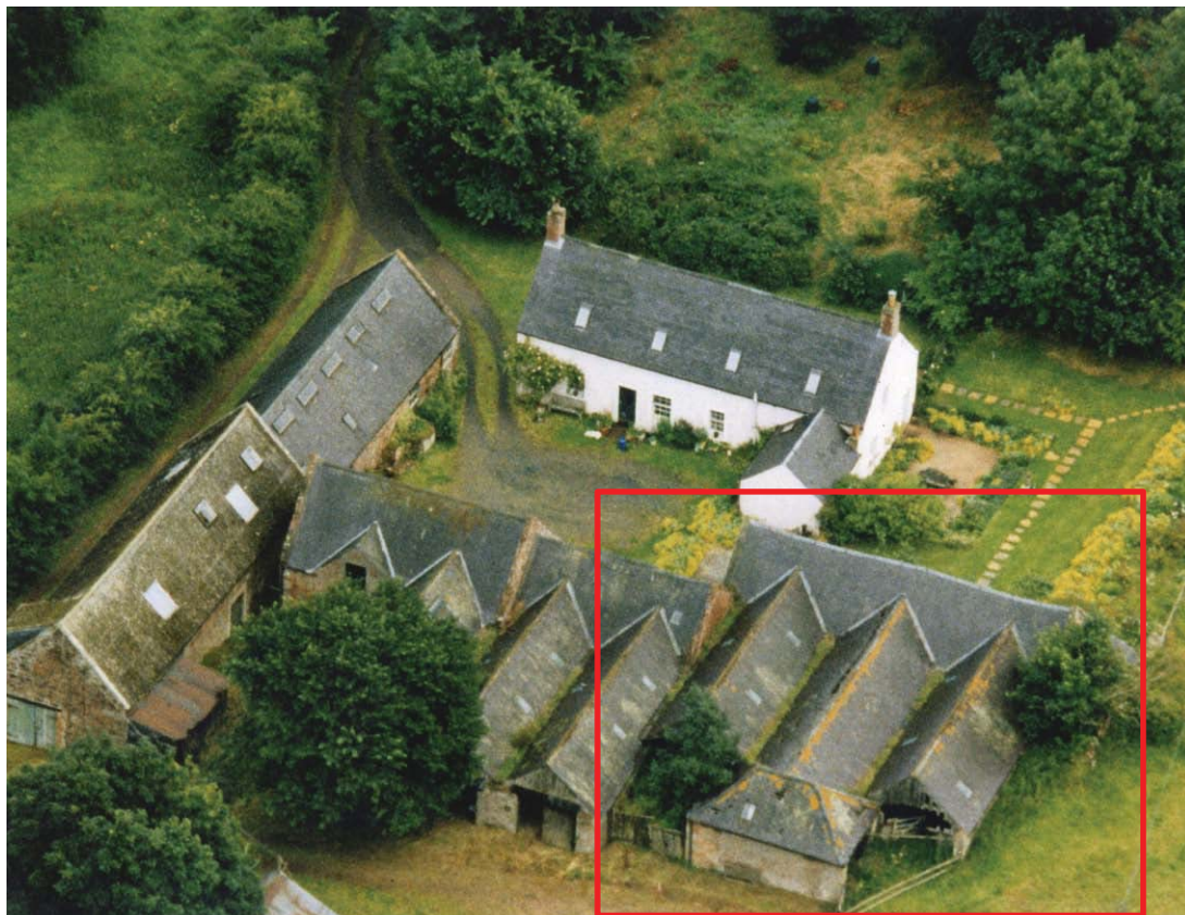
Plate 3 - A circa 1998 oblique aerial photograph of Polwarth Steading prior to the conversion of the outbuildings. The double M-shaped roof arrangement can be seen on the west side of the barn
