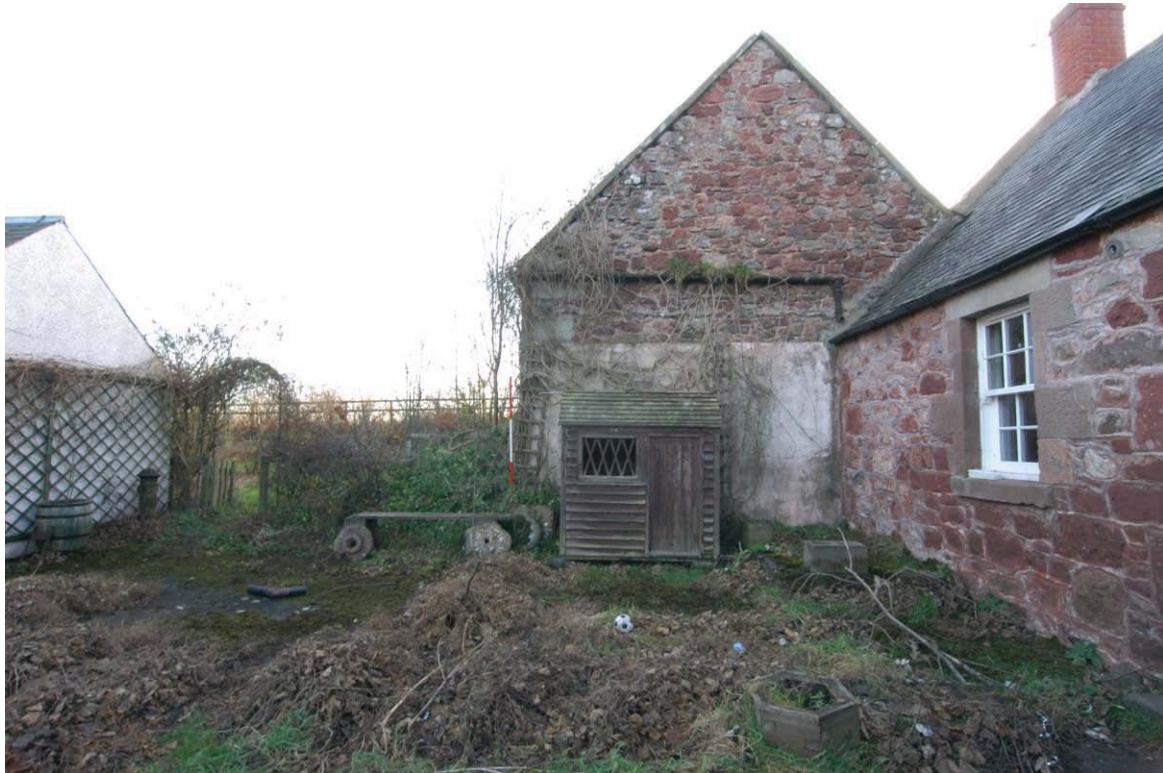
Plate 4 - North-facing elevation of the barn
