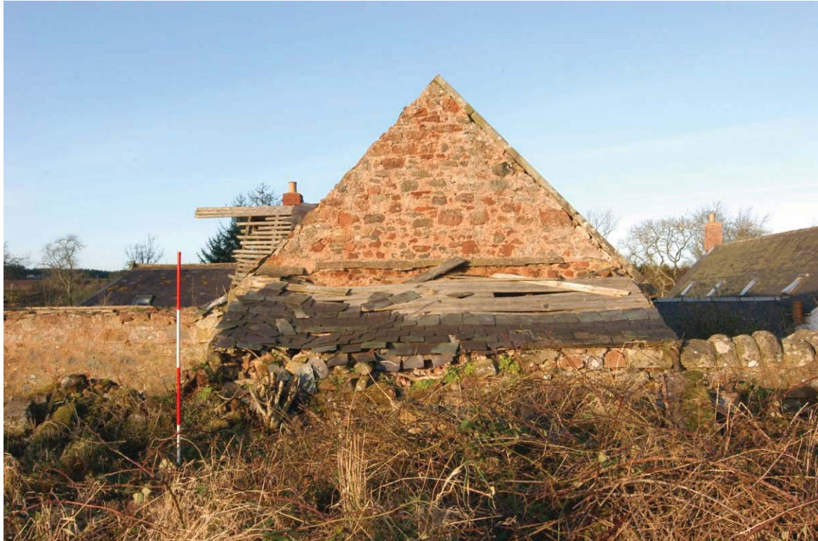
Plate 6 - South-facing gable and lean-to roof of the pigsties
