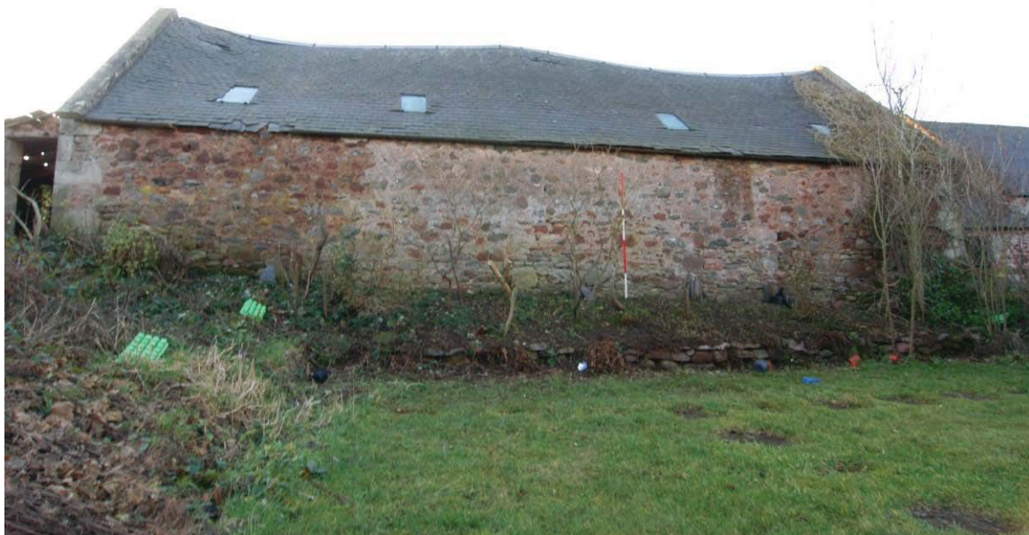
Plate 5 - East-facing elevation of the barn
