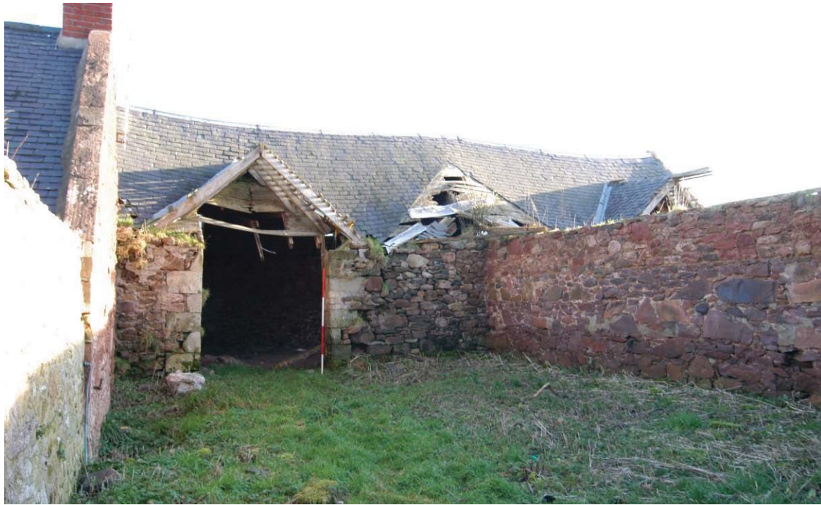
Plate 8 - Interior of the cattle court showing the entrance to Unit 1
