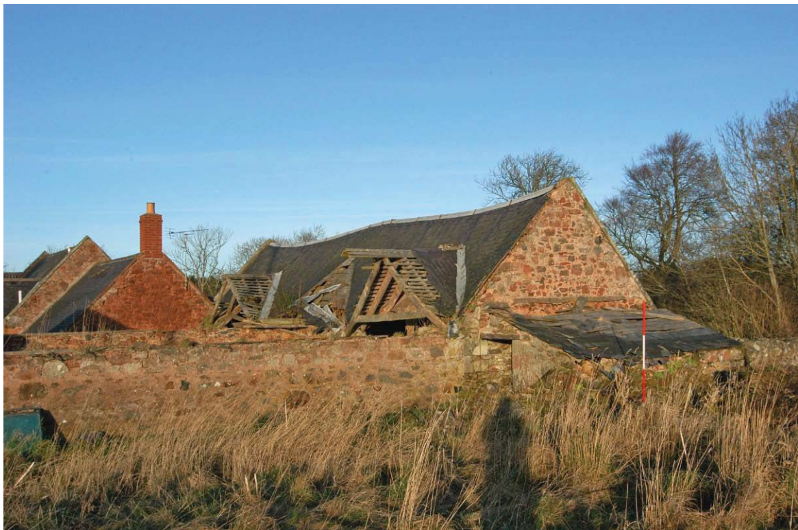
Plate 7 - General view of the west-facing elevation and south gable
