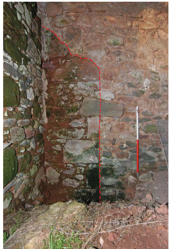
Plate 10 - Quoins of the adjoining stable block keyed into the fabric of the gable of the barn
