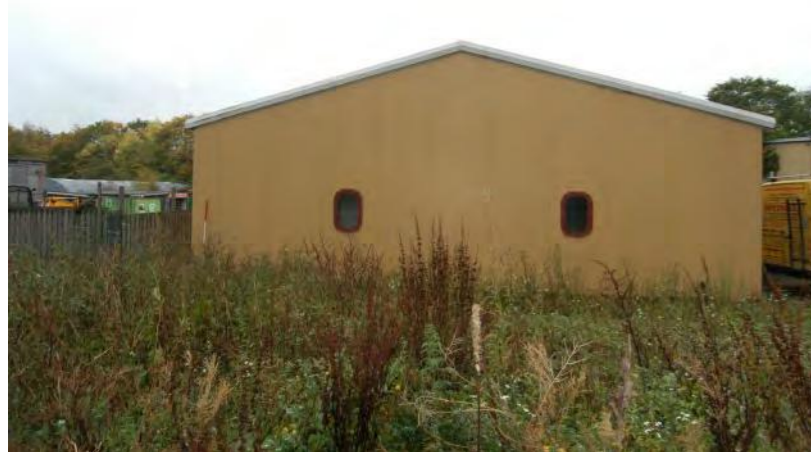
Plate 1 - Building 1, north-facing gable end (William Wilson electrical suppliers)
