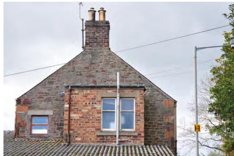
Plate 5 - Building 2, east-facing gable showing rebuilt stack and bathroom extension
