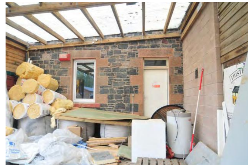
Plate 6 - Building 2, ground floor entrance with adjoining workshops
