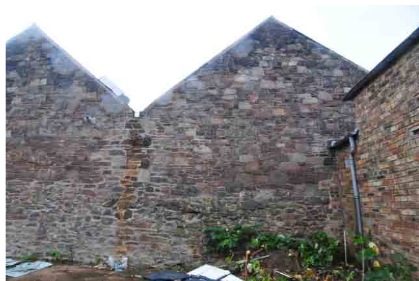
Plate 10 - Building 3, south-facing elevation, M-shaped roof arrangement and adjoining modern toilet block at east end
