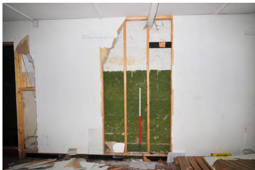
Plate 19 - Building 4, Unit 38, exposed painted wall fabric behind modern cladding
