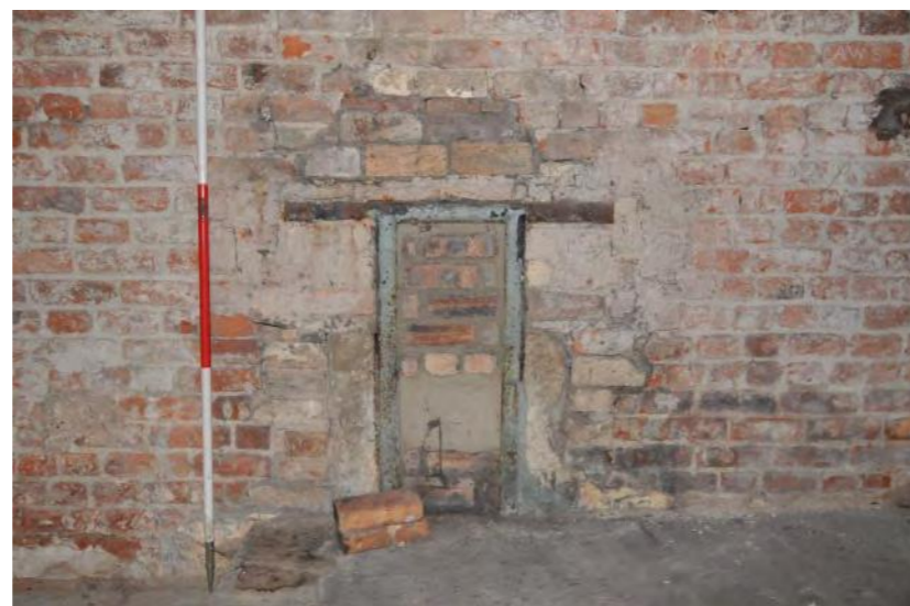
Plate 32 - Stow Station House, Unit 9, detail of coal chute
