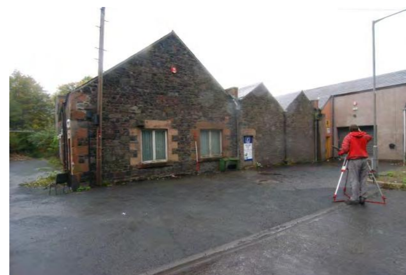
Plate 15 - Building 4, north-east facing elevation
