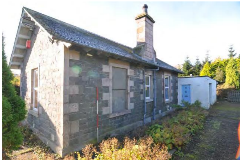
Plate 36 - Stow Station House, north-facing elevation from the north-east
