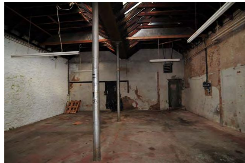
Plate 17 - Building 4, Unit 41, two replacement columns supporting the roof plate
