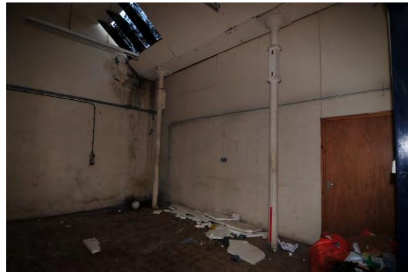
Plate 14 - Building 3, Unit 28 two cast-iron columns with holes for line-shaft brackets
