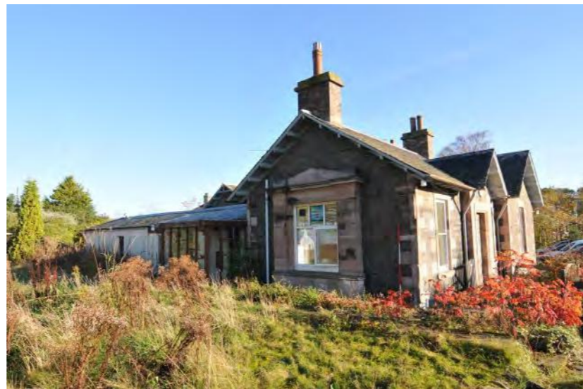
Plate 40 - Stow Station House, west-facing elevation from the south-west
