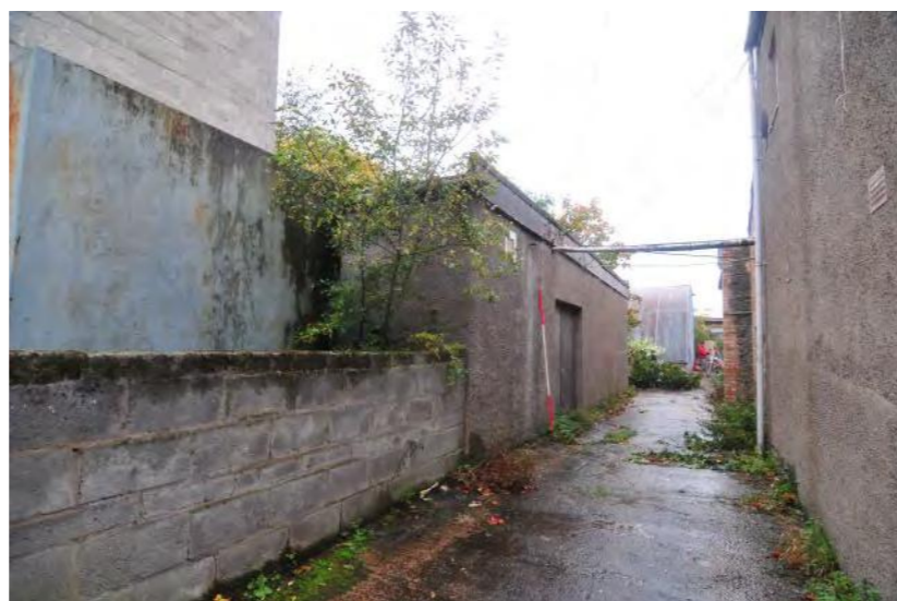
Plate 23 - Building 5, Unit 3 north-facing elevation of the main plant room
