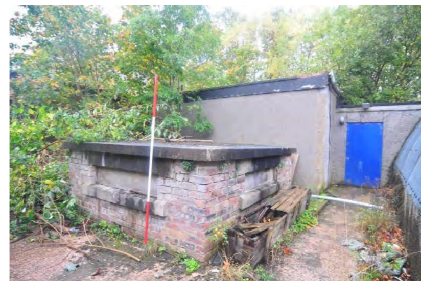
Plate 24 - Building 5, Unit 2 engine house, north and west-facing elevations
