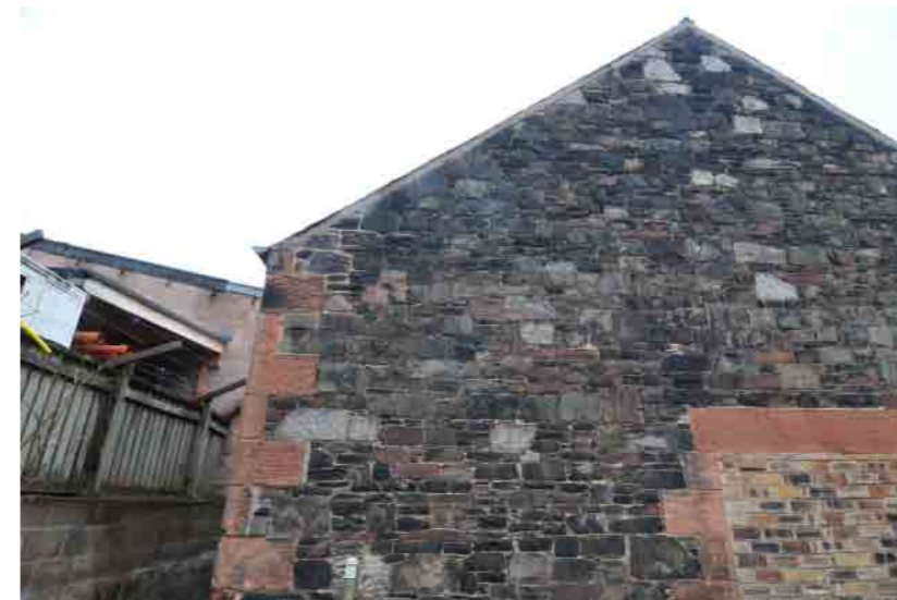
Plate 9 - Building 3, south-facing elevation, fabric detail and blocking work
