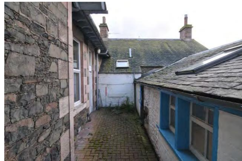
Plate 41 - Stow Station House, view of the yard from the north
