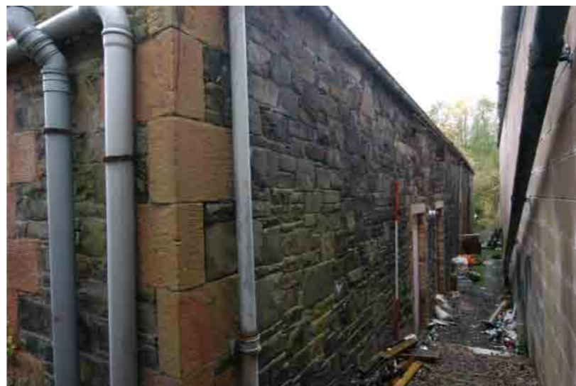
Plate 8 - Building 3, west-facing elevation and the east-facing elevation of Fjordhus workshops
