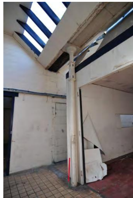
Plate 13 - Building 3, Unit 28 a cast-iron column with sockets for a line-shaft bracket
