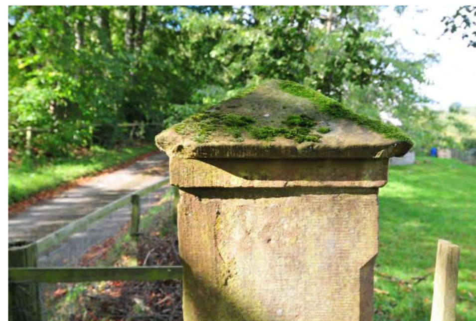
Plate 45 - Torwoodlee Gate Piers, detailed shot of the pyramid-shaped coping stone
