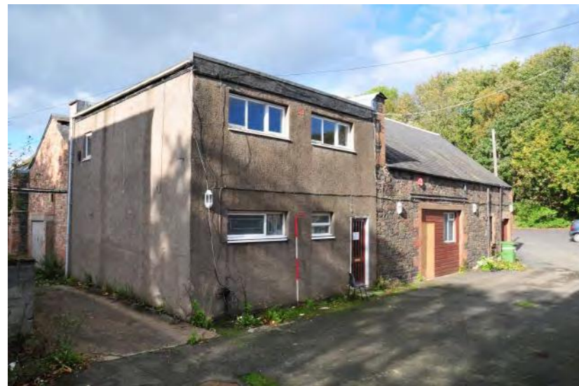
Plate 16 - Building 4, east and south-facing elevations
