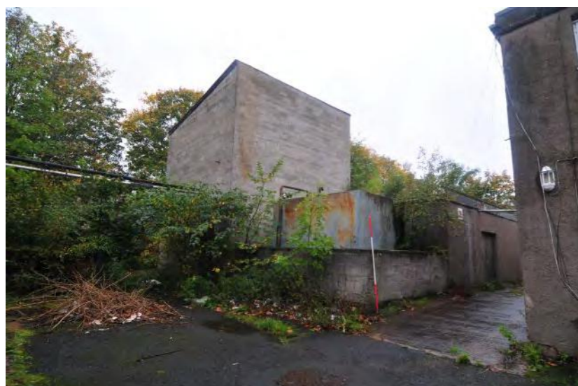
Plate 22 - Building 5, Unit 22 north-facing elevation of the shuttered concrete building
