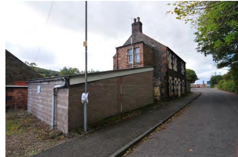
Plate 3 - Building 2, north and east-facing elevations of the former Fjordhus Ltd offices
