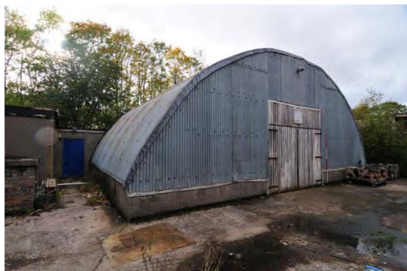
Plate 20 - Building 5, Unit 1 north-facing elevation
