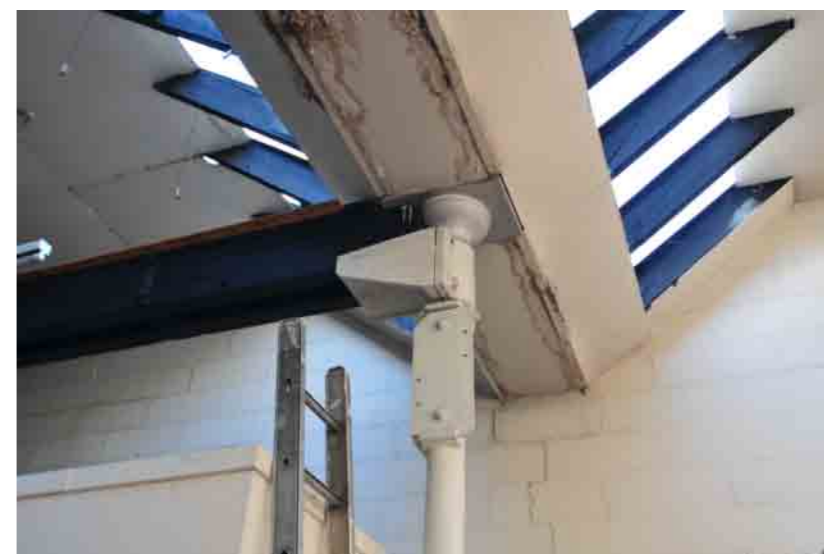
Plate 12 - Building 3, Unit 33 cast-iron column head with holes for line-shaft bracket
