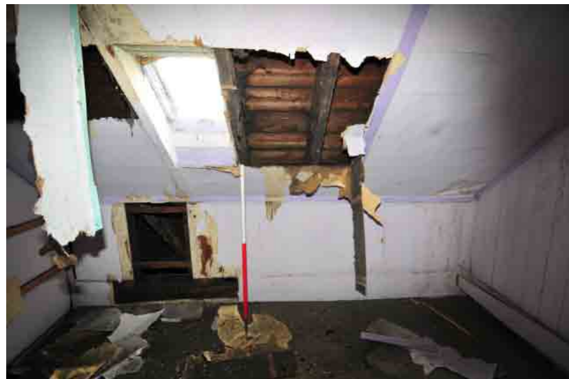
Plate 7 - Building 2, exposed roof truss and sarking boards in Unit 20
