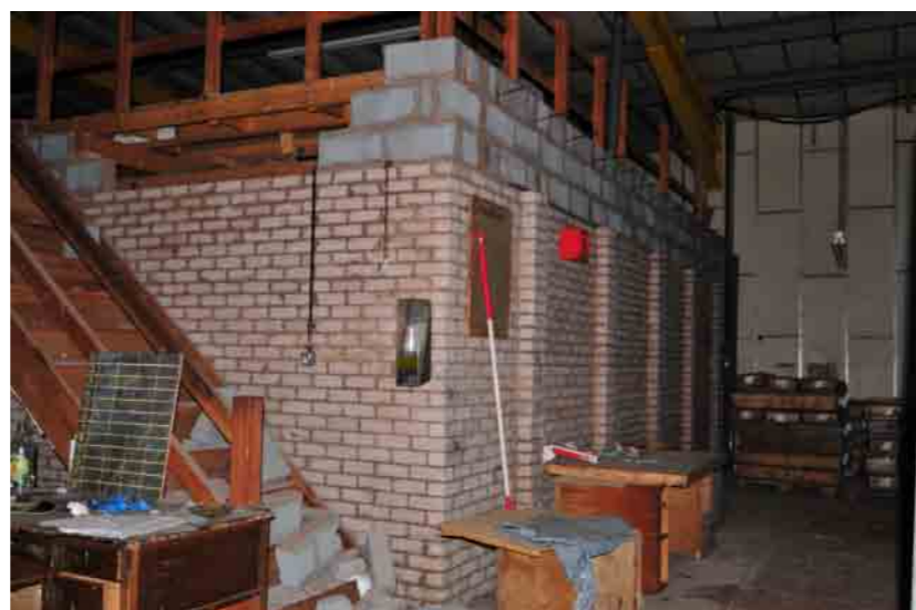
Plate 29 - Building 6, Unit 2 exterior east-facing wall and staircase to mezzanine floor
