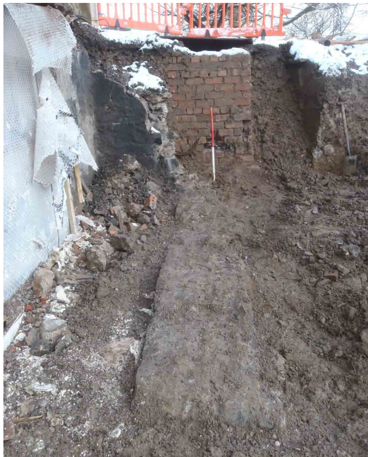
Fig. 6 - The wall (045) beneath the conservatory with septic tank in the background
