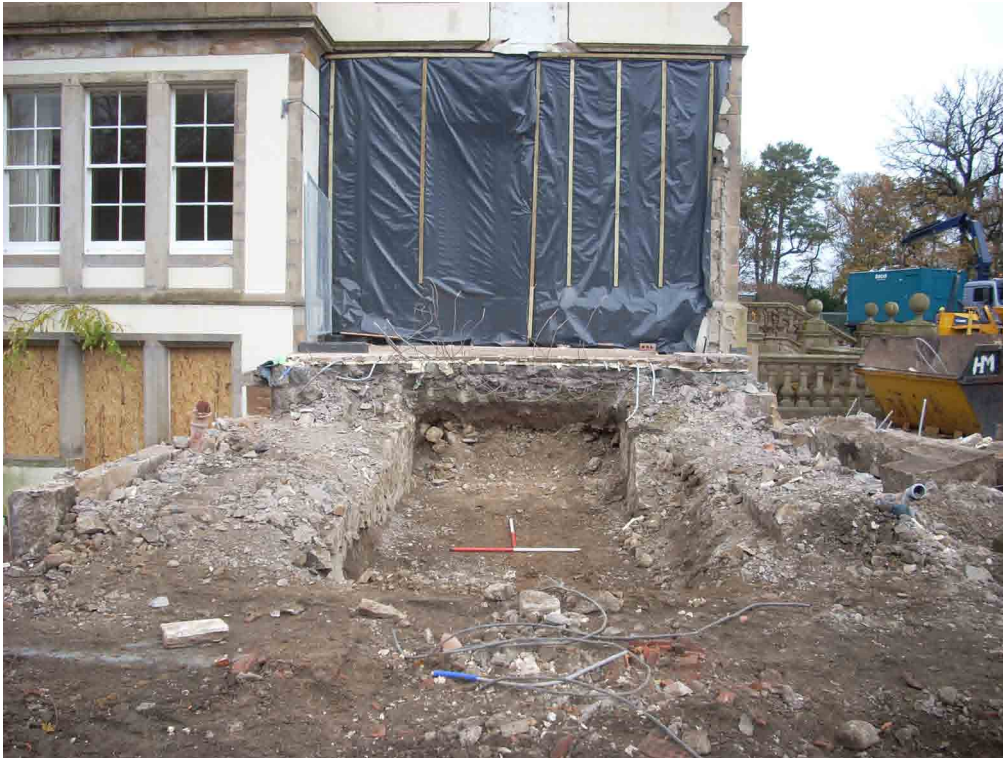
Fig. 3 - The footings beneath the demolished conservatory
