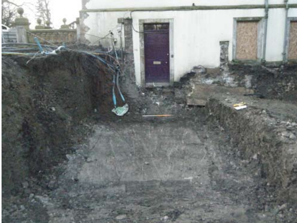
Fig 7 - The demolished boiler house with concrete floor (053) visible
