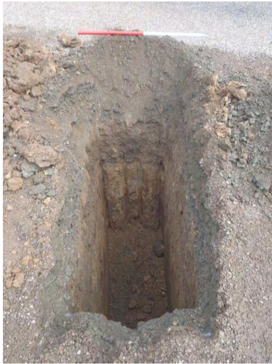
Fig. 5 TP 2, post excavation
