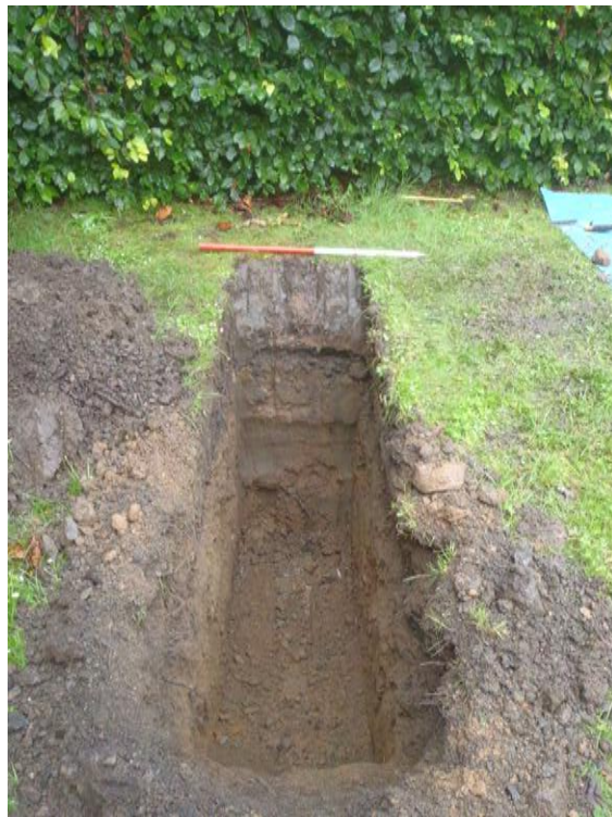
Fig. 6 TP 3, post excavation
