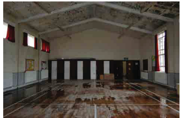
Fig. 15 North end of the Large Hall with lockers
