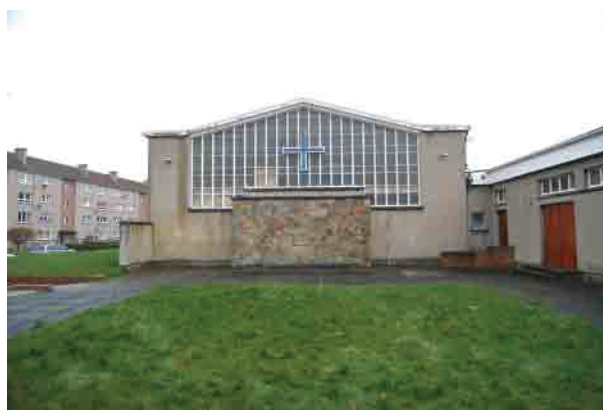
Fig. 5 West facing gable of St Martin's Church
