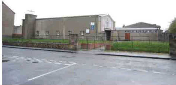
Fig. 3 North-facing elevation of St Martin's Church
