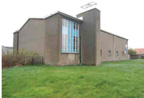
Fig. 4 North and east-facing gable wall of St Martin's Church
