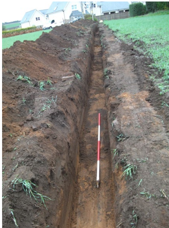
Fig. 3 Post-ex shot of cable trench from the south
