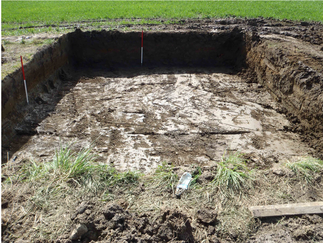
Fig. 7 - Turbine 3 fully excavated
