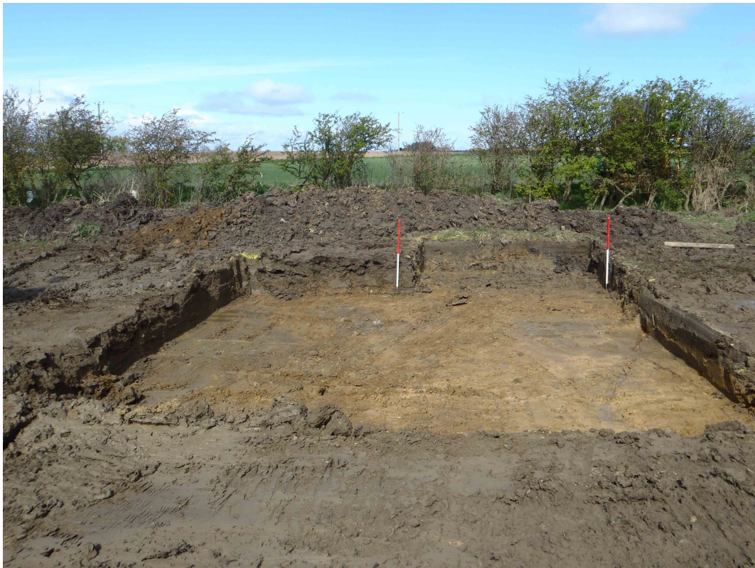
Fig. 6 - Turbine 2 fully excavated
