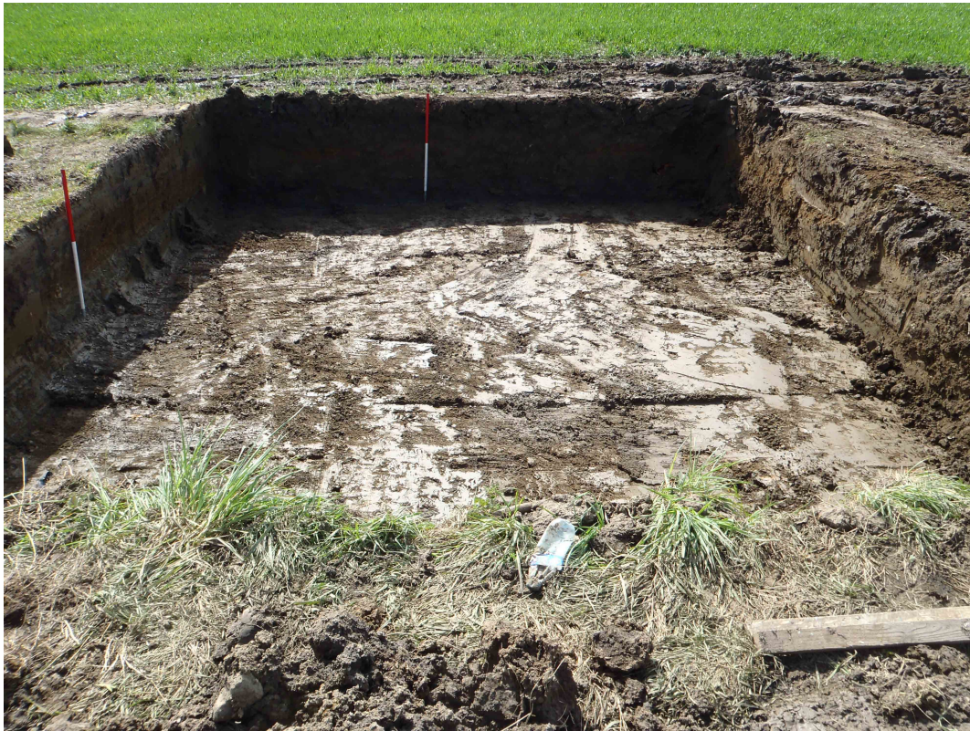
Fig. 7 - Turbine 3 fully excavated
