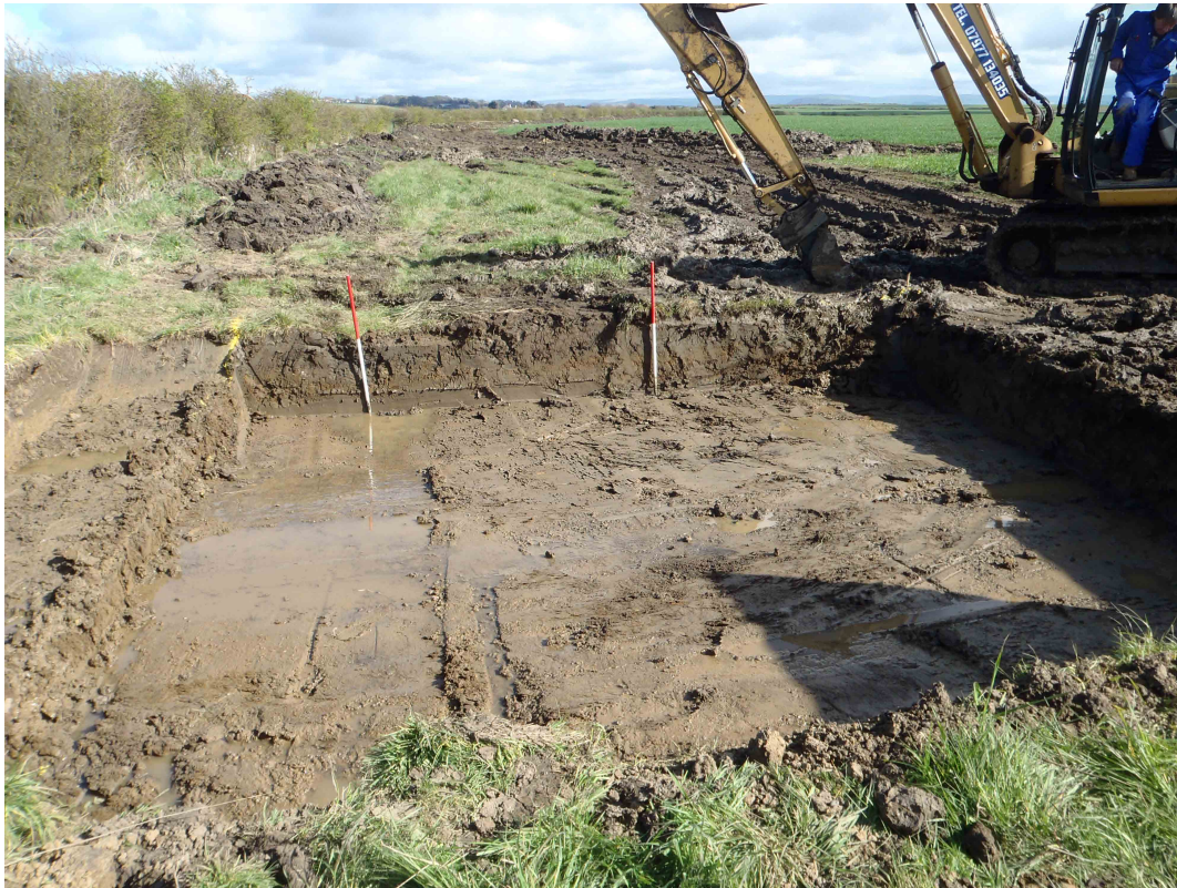
Fig. 5 - Turbine 1 fully excavated
