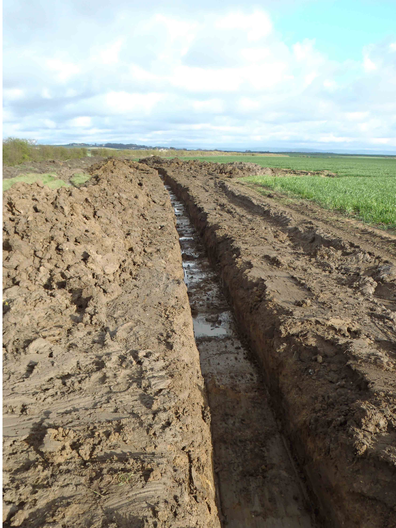
Fig. 9 - Cable Trench from NW
