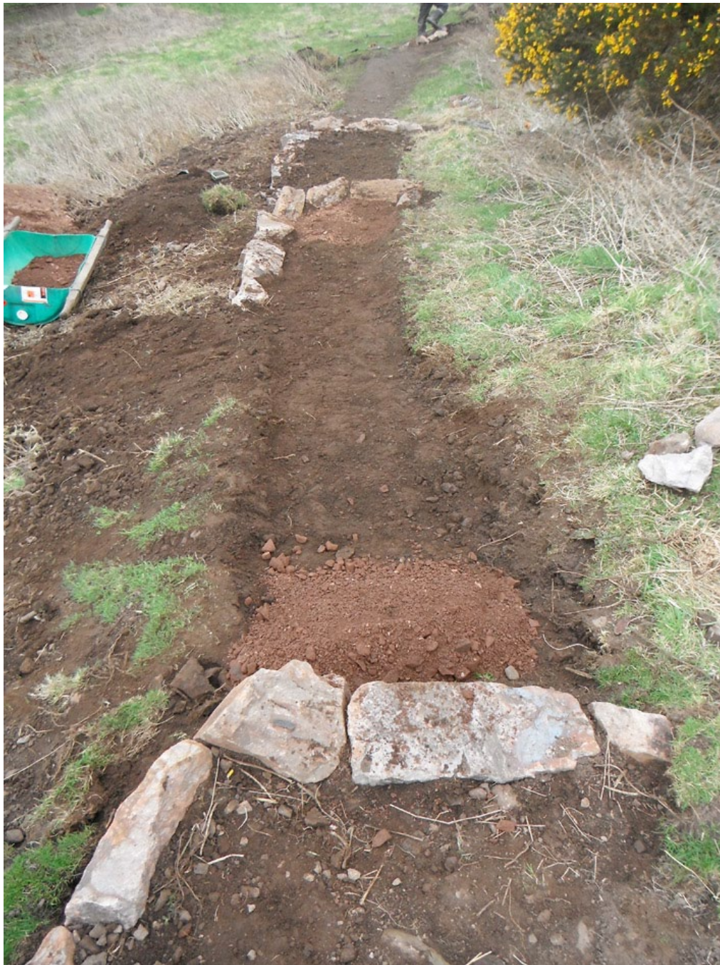
Fig. 4 - Re-surfacing between anchor bars
