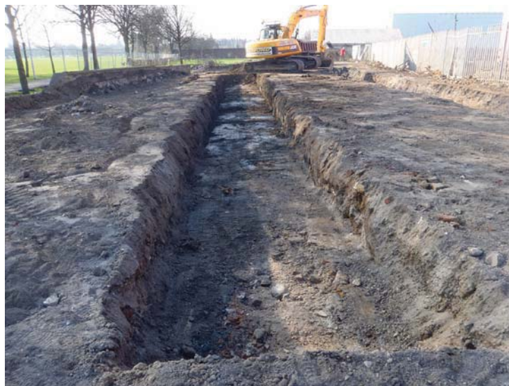
Fig. 3 - The excavated trench for one of the tensor retaining wall foundations
