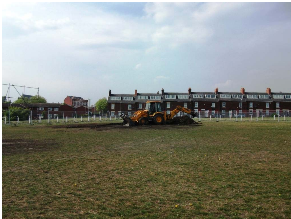
Plate 4: Backfilling the Evaluation Trenches, Looking Northwest
