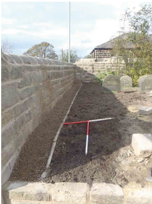
Plate 3 - Shot of Trench after backfilling
