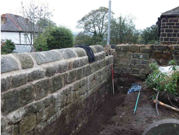
Plate 1 - Shot of excavated trench for French drain
