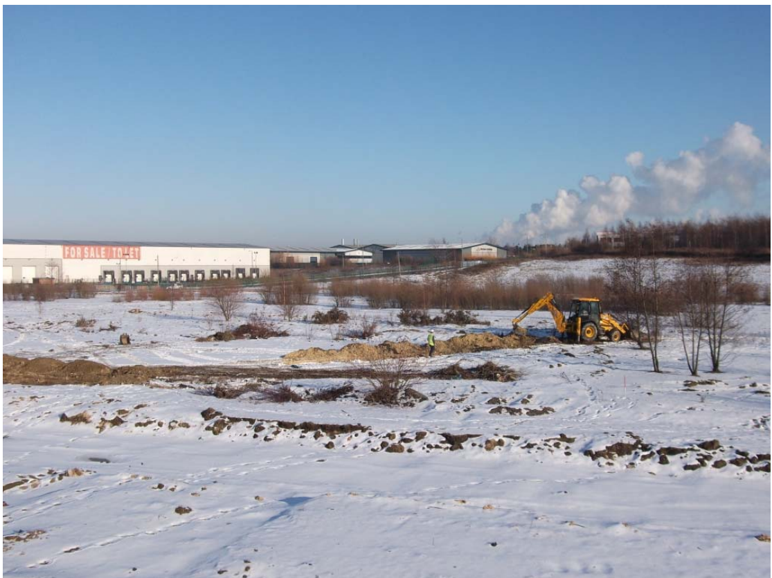
Plate 2: General Site Shot, Looking Northwest
