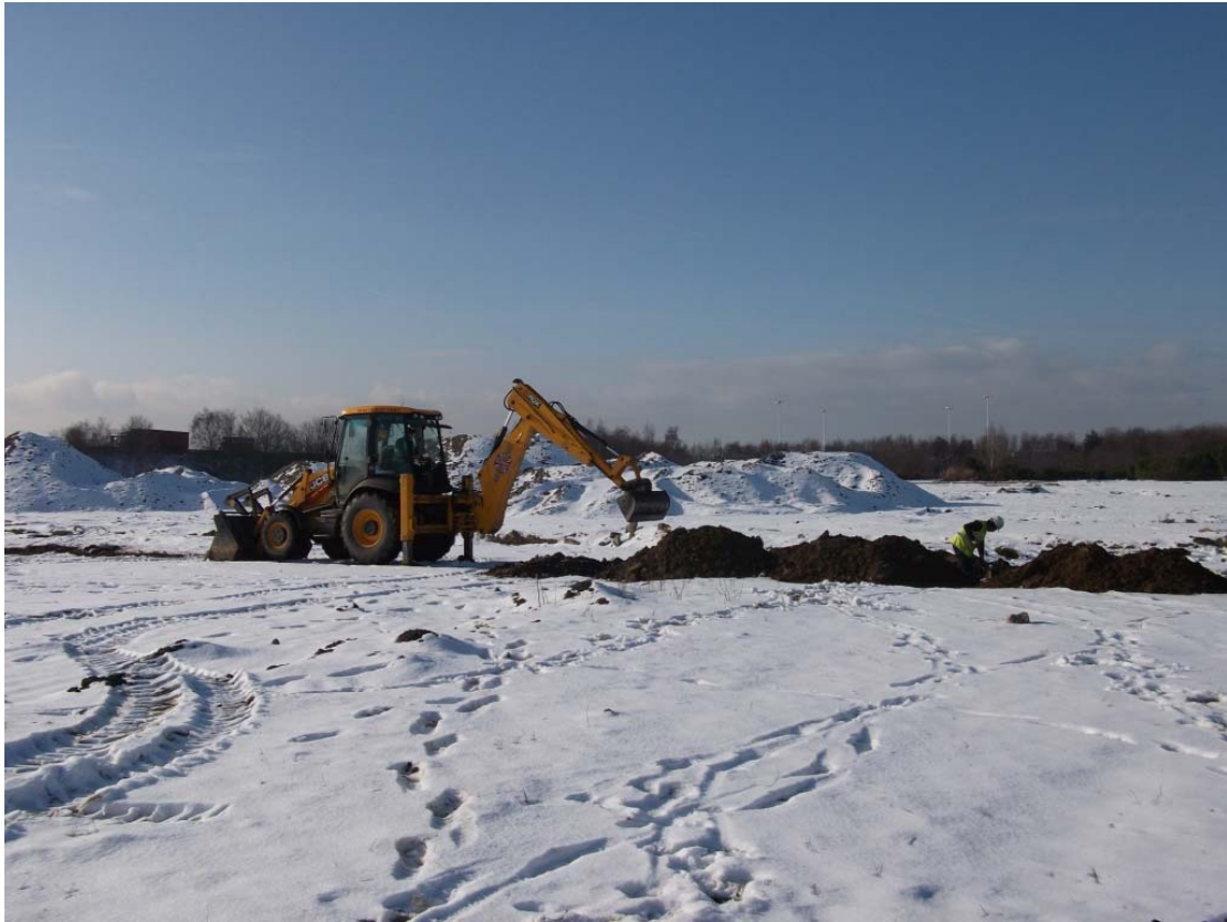
Plate 3: Working Shot during the Excavation of Trench 2
