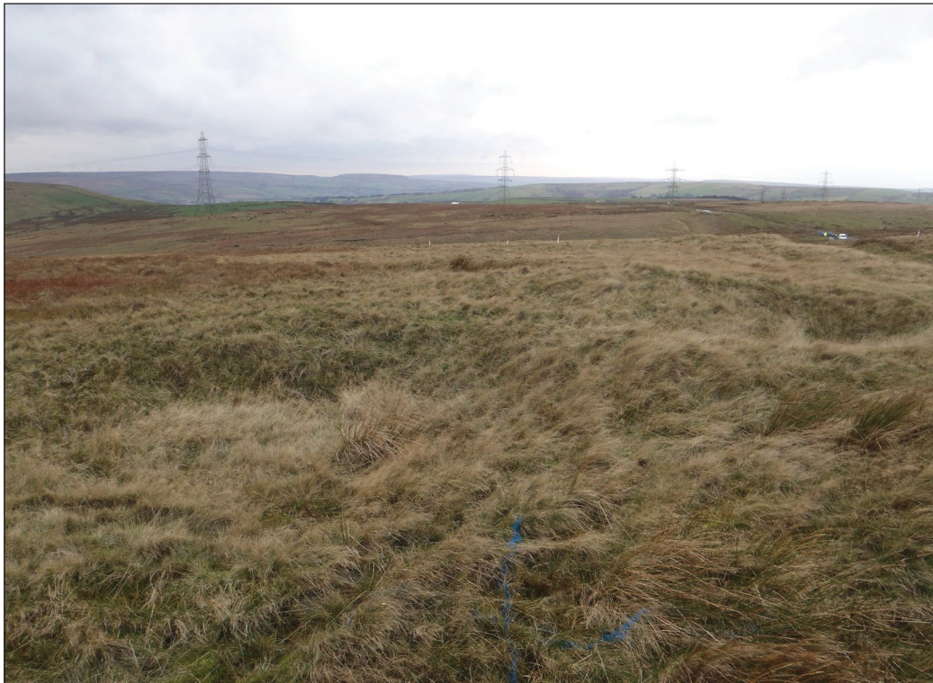
Figure 8 - General shot overlooking Turbine 3 access road
