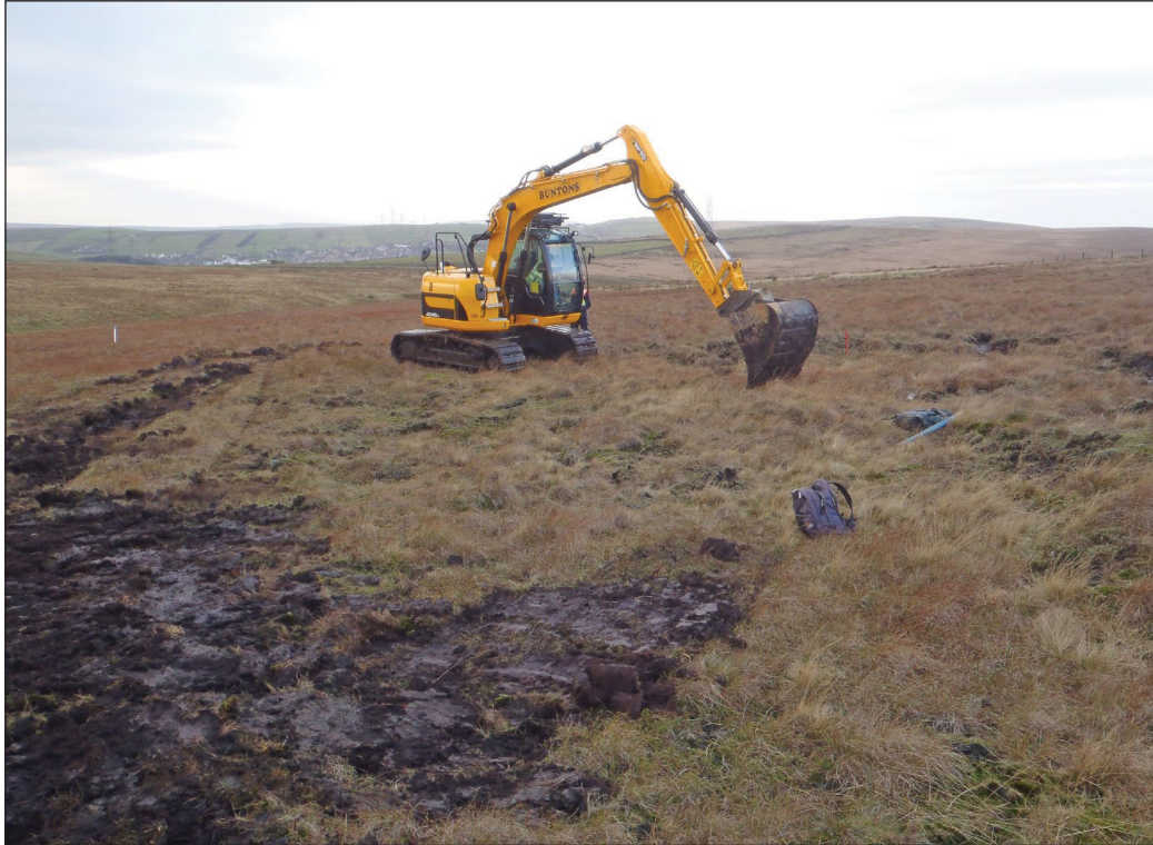
Figure 9 - Working shot of conditions during test-pit excavation
