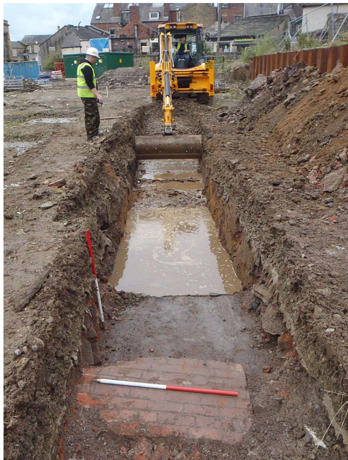
Fig. 6 - Working Shot of Trench 1 Excavation and Surface (103)
