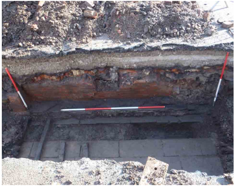
Fig. 8 - Shot of West-Facing Section of Trench 2; Walls (206 & 207); Surfaces (213 & 215)
