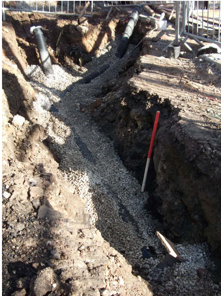
Fig. 20 - Post-excitation Shot of Trench B in Watching Brief Area
