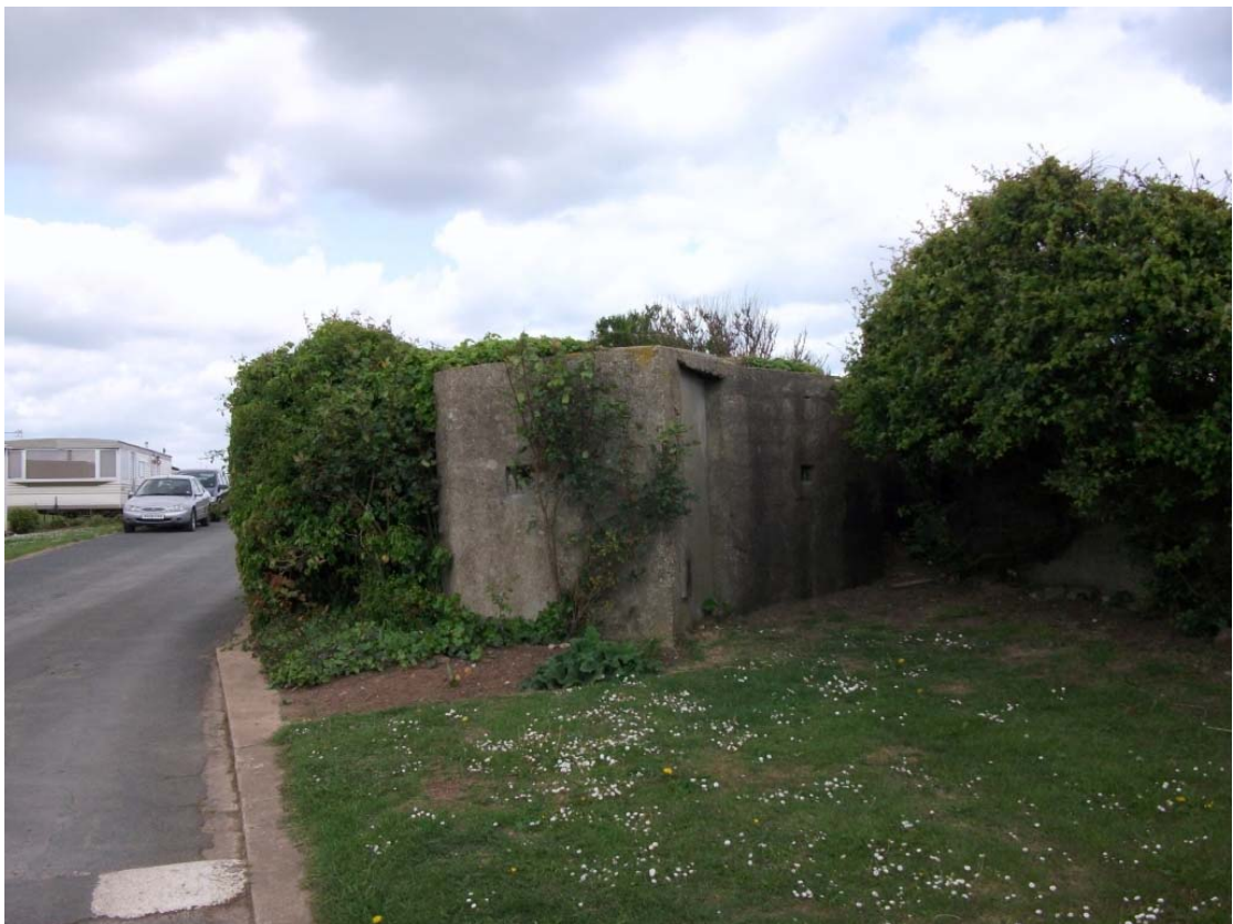
Plate 6: Coastal Pillbox on the Edge of Sand-le-Mere Caravan Park
