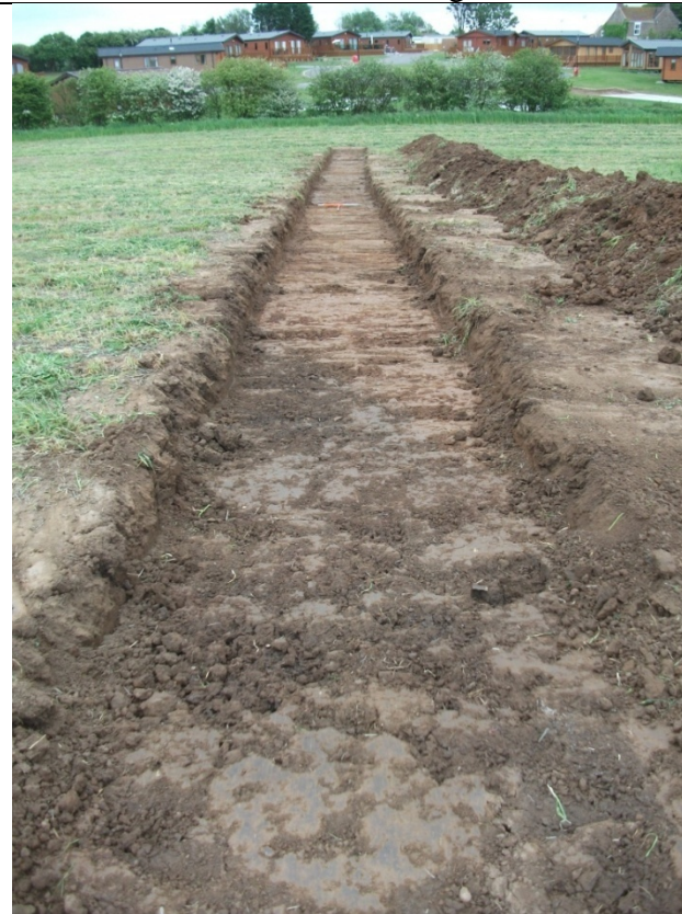
Plate 1g: Trench 9 Looking Southwest
