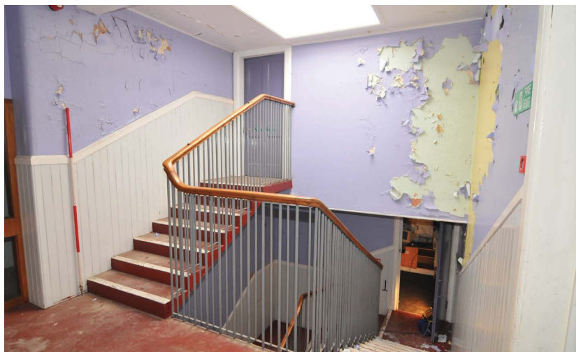
Plate 16 - Unit 20 - Top of stairs and landing
