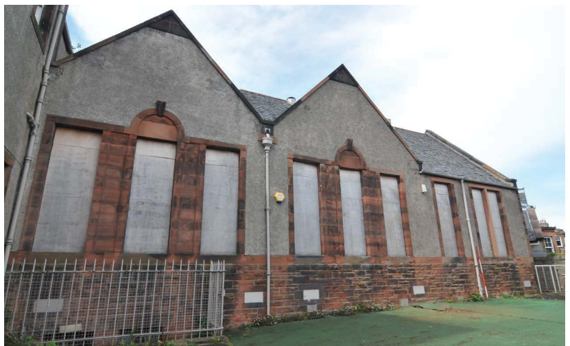
Plate 4 - SE facing elevation, central block
