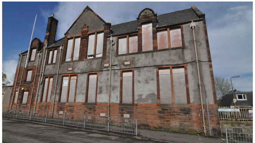
Plate 2 - SW facing elevation, south block
