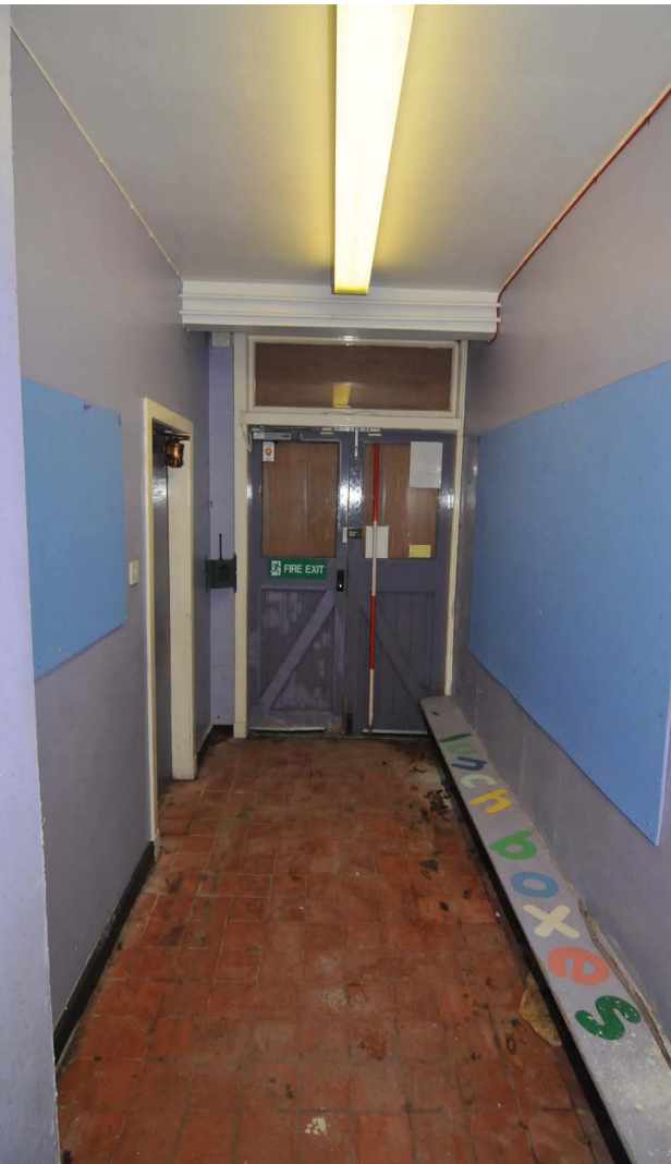
Plate 10 - Unit 7 - Entrance corridor
