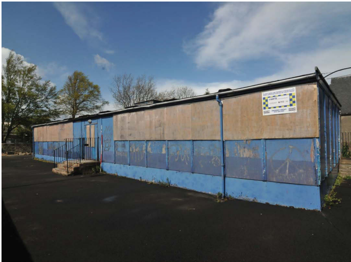
Plate 7 - General view of prefabricated building
