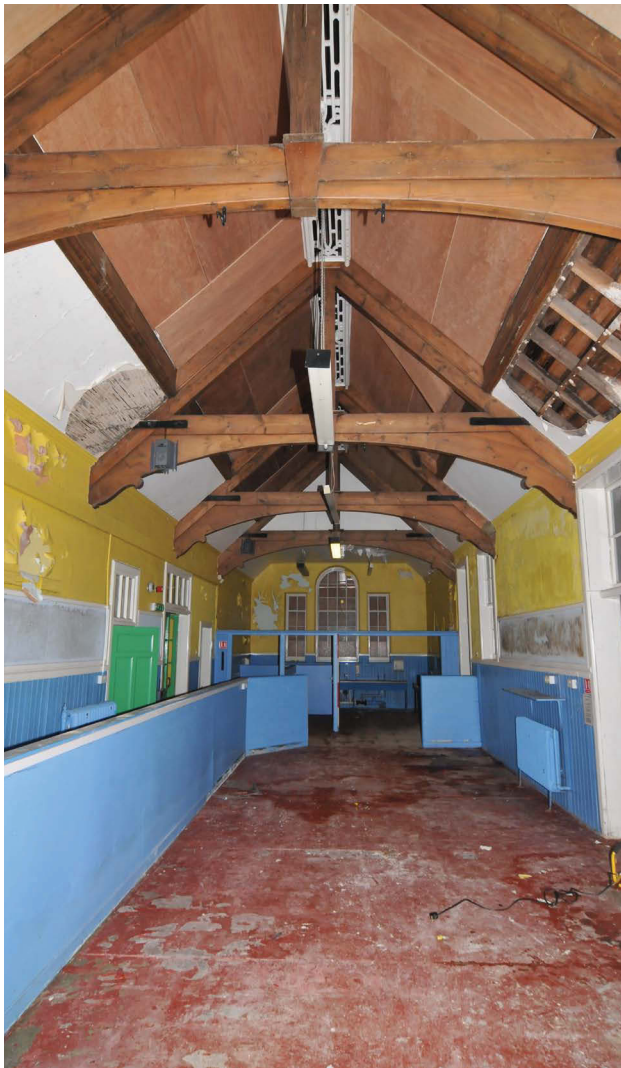
Plate 15 - Unit 17 - Main hall and roof truss
