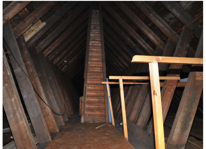
Plate 20 - Unit 21 - Rooftruss and timber chimney vent
