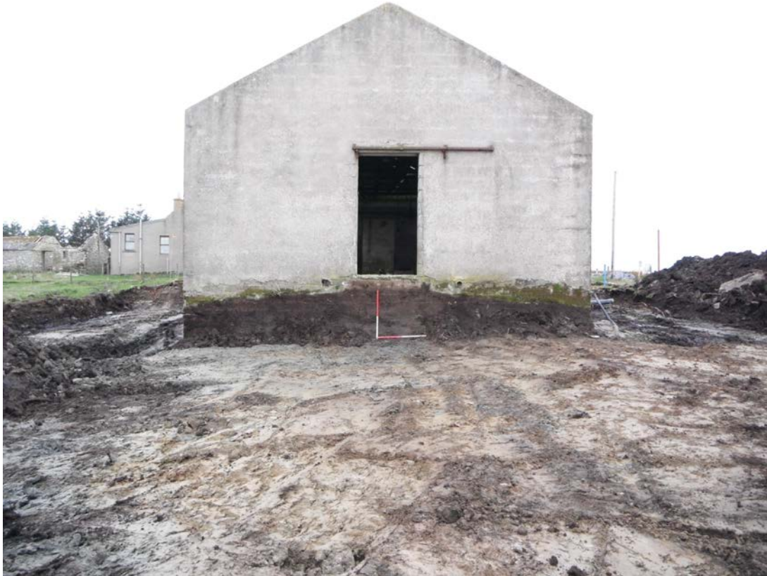
Fig. 8 - Topsoil stripping at Badlipster Farm
