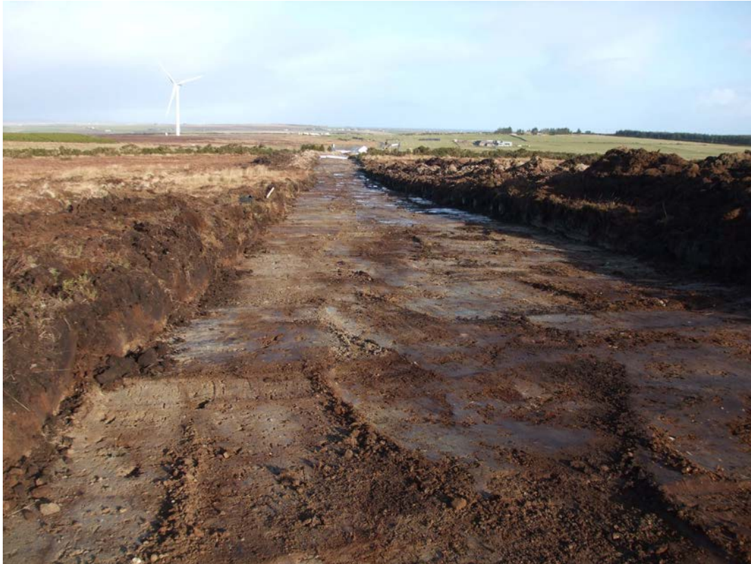
Fig. 4 - General vie of topsoil stripping along principal access track from Achairn
