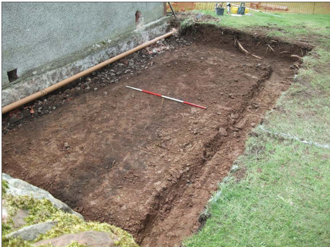
Fig. 3 - Watching brief area following excavation. From the north.
