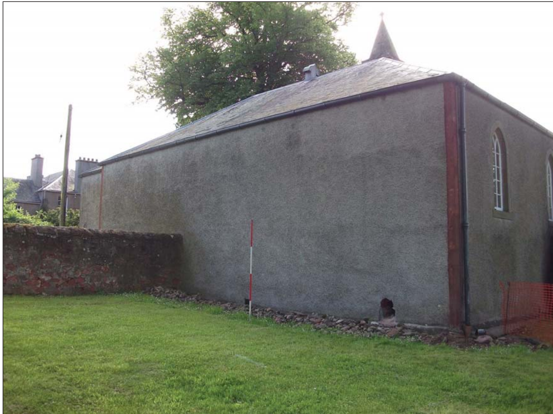
Fig. 2 - Watching brief area prior to excavation. From the west.
