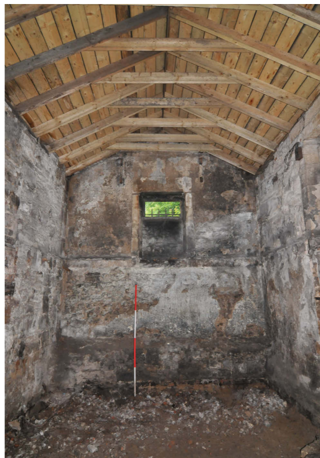
Plate 8 - Interior, east-facing elevation showing floor joists
