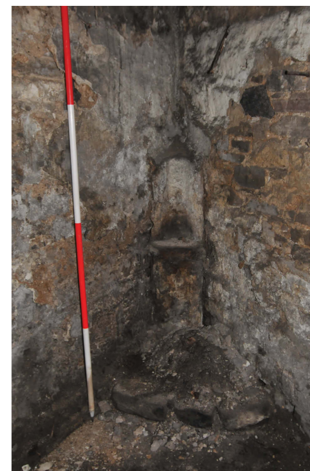
Plate 12 Interior, corner of west and south-facing elevation
