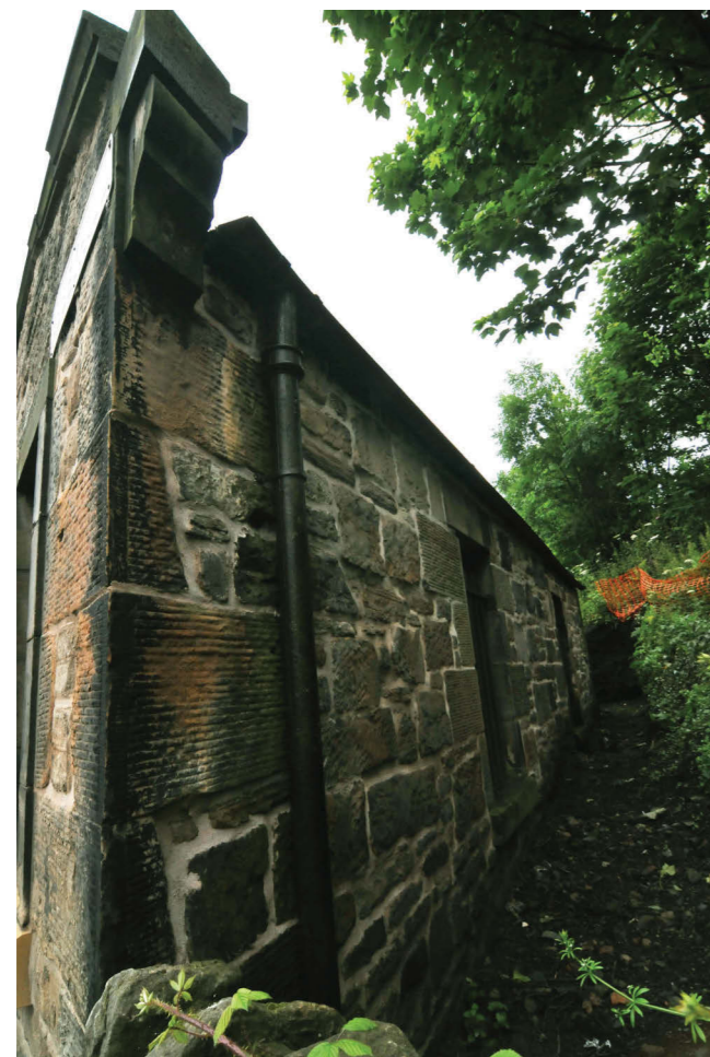
Plate 4 - Exterior, oblique view of the north-facing elevation
