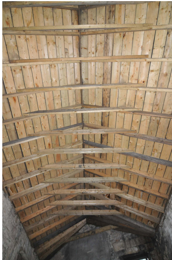
Plate 14 - Interior roof trusses and sarking boards
