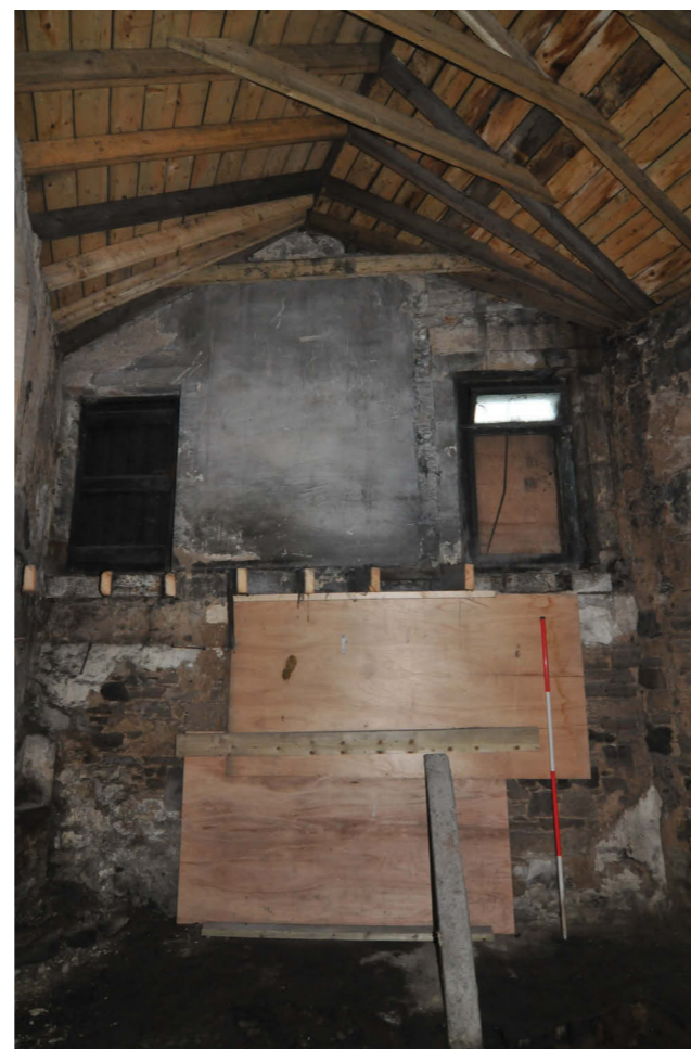
Plate 5 - Interior, west-facing elevation
