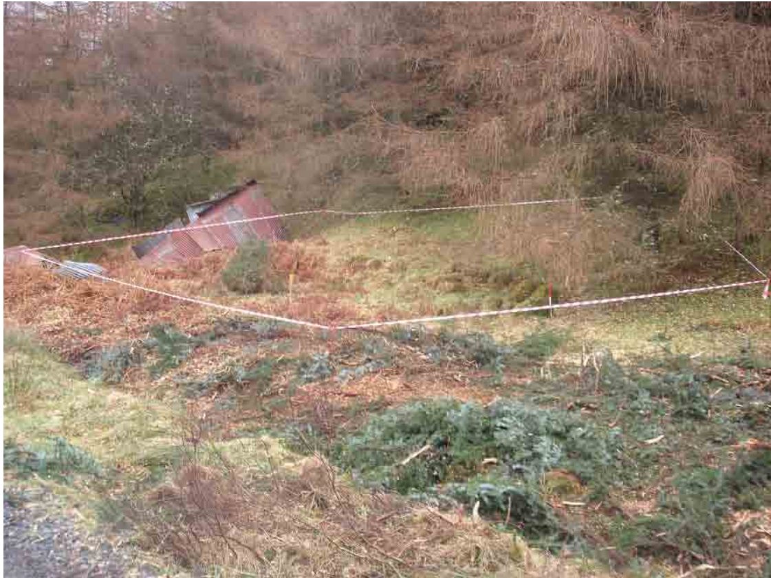
Fig 40 - Shot of Site CFA 6 during demarcation works
