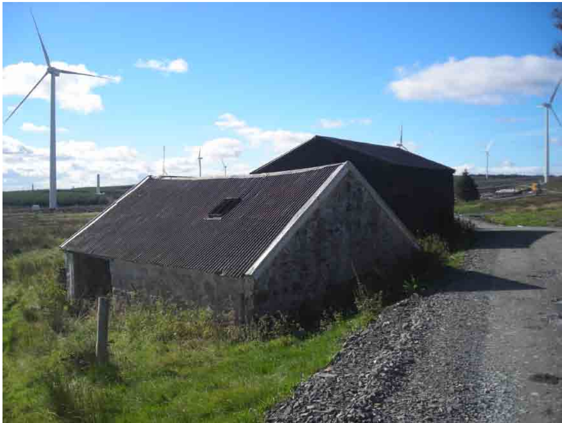
Fig 25 - Shot of Site 83 east during demarcation works
