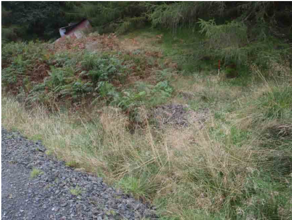
Fig 41 - Shot of Site CFA 6 after wind farm construction
