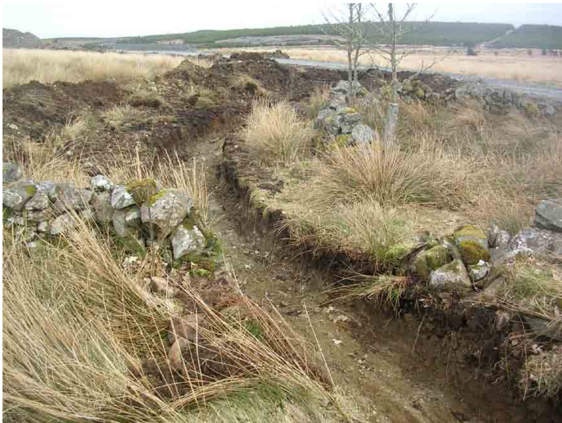
Fig 27 - Shot of Site 83 during watching brief on cable trenching
