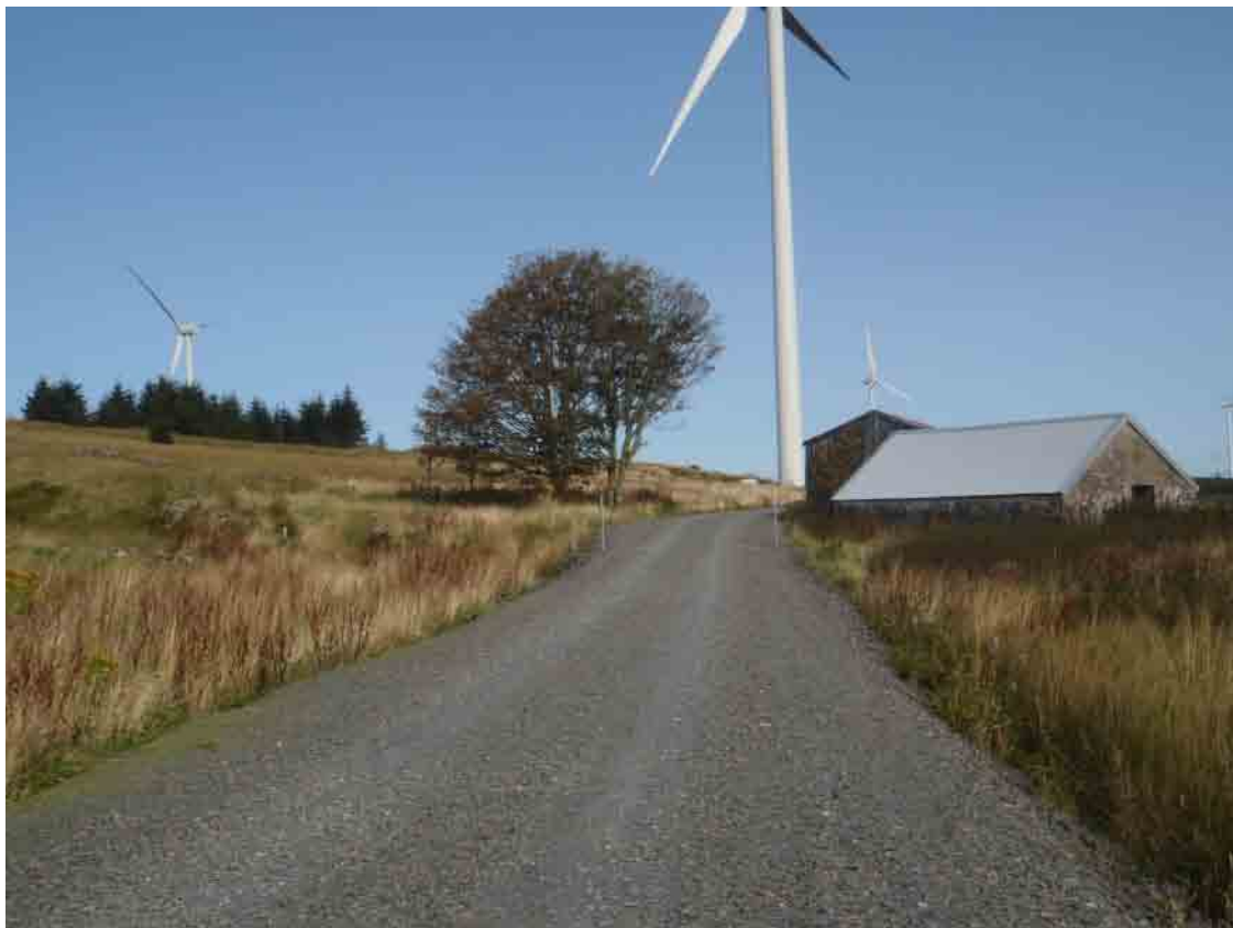
Fig 37 - Shot of Site 83 after wind farm construction
