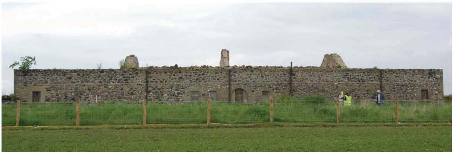
Fig. 16 - General view of the exterior north-facing elevation
