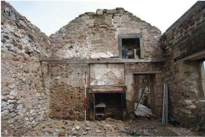
Fig. 5 - Unit 1, interior west-facing elevation showing two fireplaces
