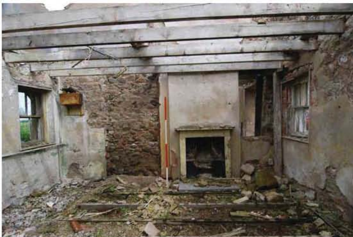
Fig. 7 - Unit 2, interior west-facing elevation showing the fireplace
