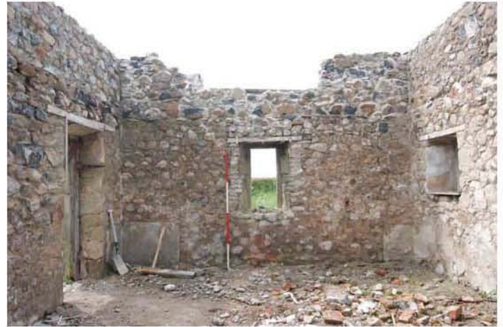
Fig. 6 - Unit 1, interior east-facing elevation showing the gable wall
