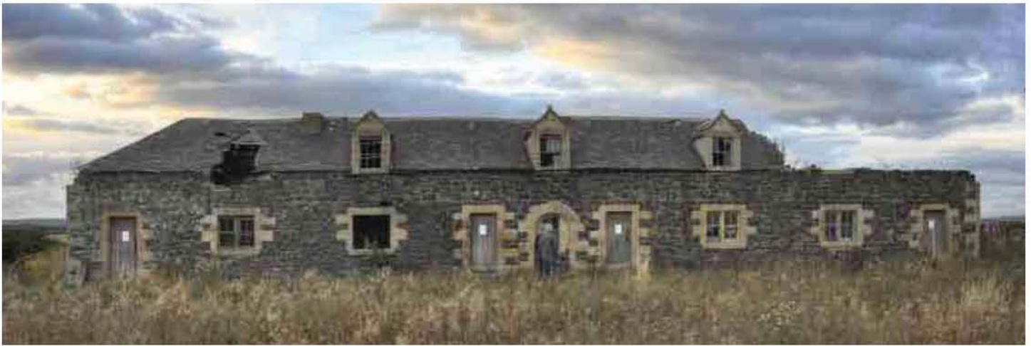
Fig. 17 - General view of the exterior south-facing elevation prior to roof removal
