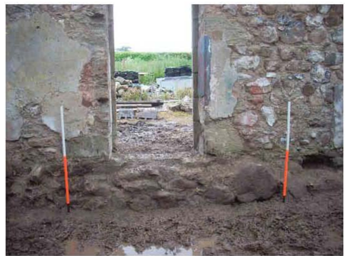
Fig. 22 - Exposed foundations in Unit 2 during the watching brief
