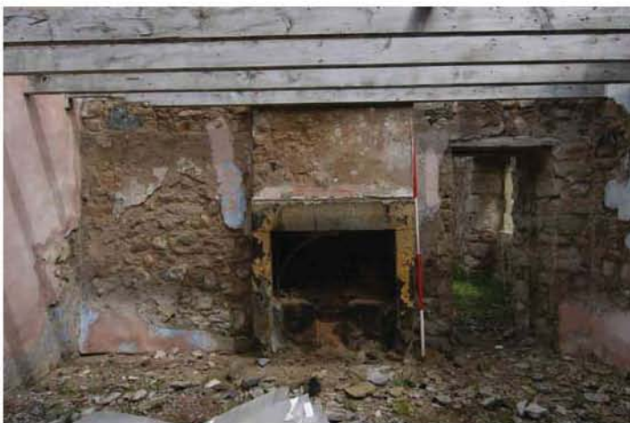
Fig. 9 - Unit 3, interior west-facing elevation showing the fireplace
