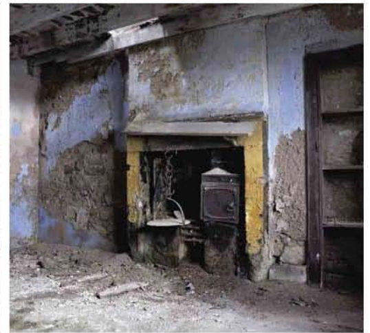
Fig. 20 - Unit 3 fireplace prior to stripping out the building
