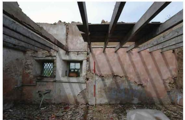
Fig. 8 - Unit 2, interior south-facing elevation showing windows
