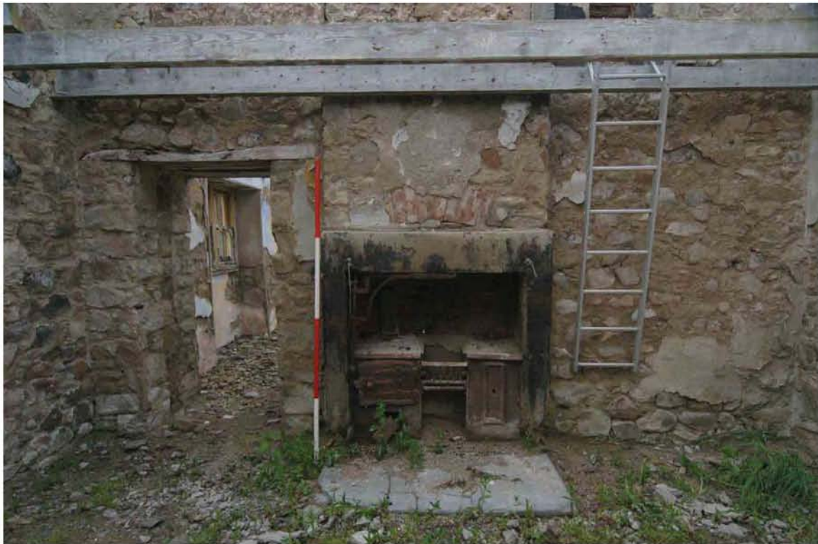
Fig. 11 - Unit 4, interior east-facing elevation showing the fireplace
