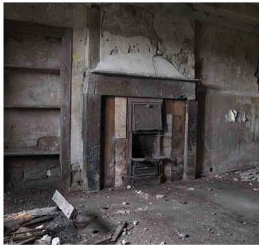
Fig. 19 - Unit 2 fireplace prior to stripping out the building
