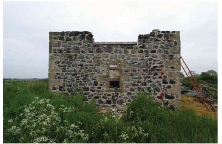
Fig. 15 - General view of the exterior west-facing gable
