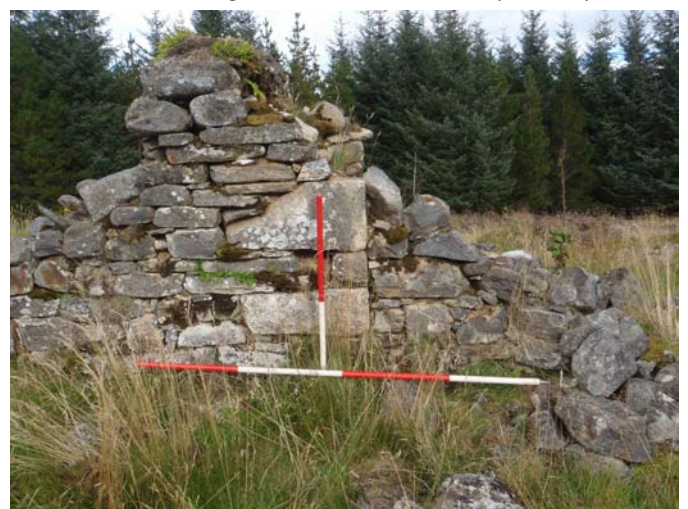
Fig. 20 - Shot of quoining where Room 6 abuts Room 5 (Site 1a)
