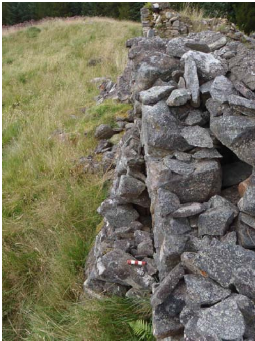
Fig.21 - Detailed shot of drystone buttressing against west wall of Room 5 (Site 1a)
