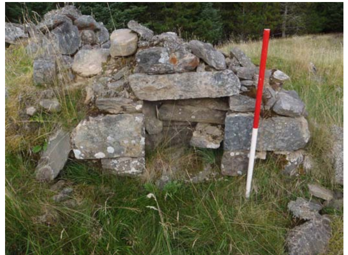
Fig.18 - Shot of blocked feature/ probable window in external west-facing elevation of Room 6 (Site 1a)
