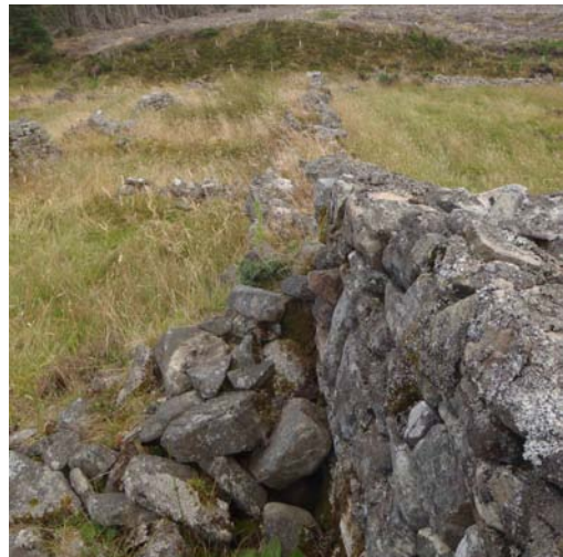
Fig.12 - General shot of offset wall alignment of Room 1-4 with Room 5 in foreground (Site 1a)
