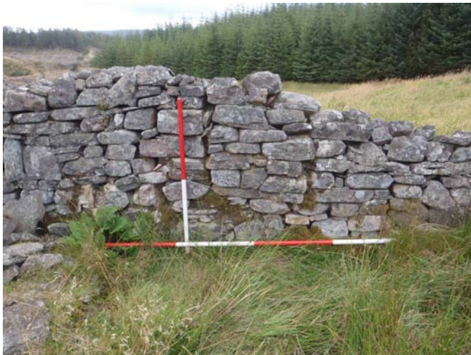
Fig.11 - Detailed shot of blocked opening & probable window Room 5 (Site 1a)
