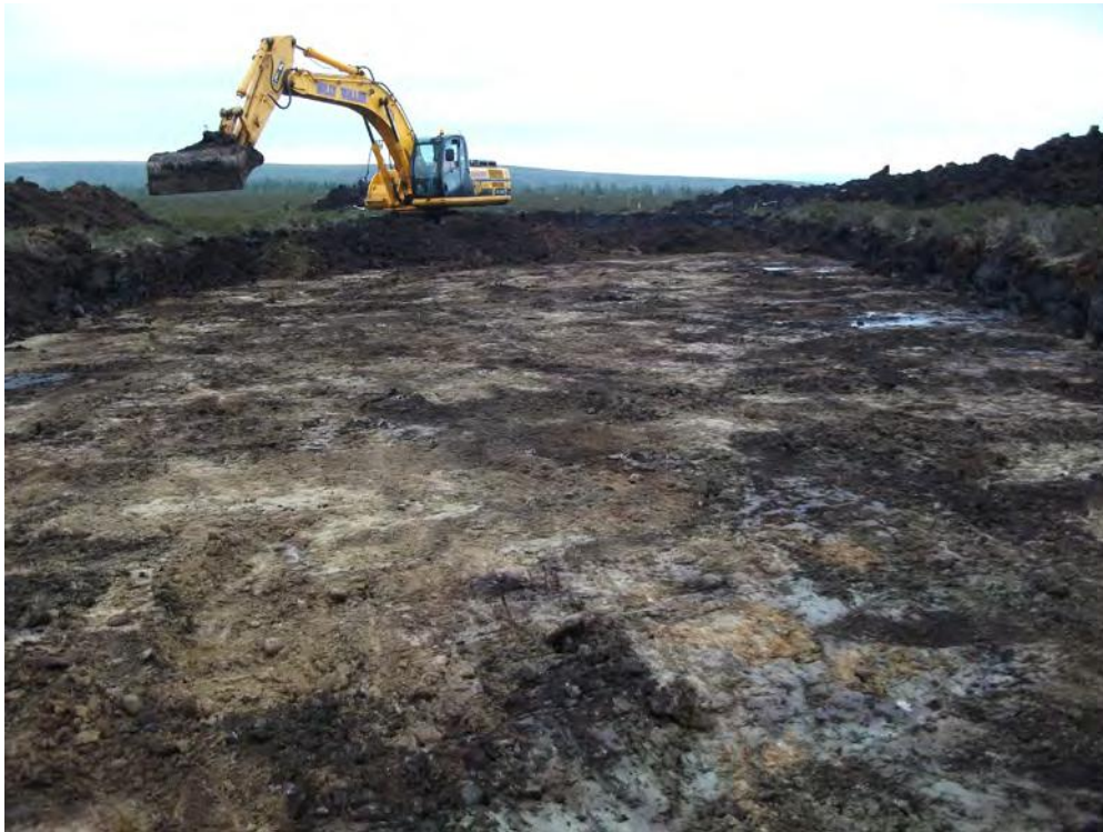
Fig. 7 Removing topsoil on access track to Turbine Base 6
