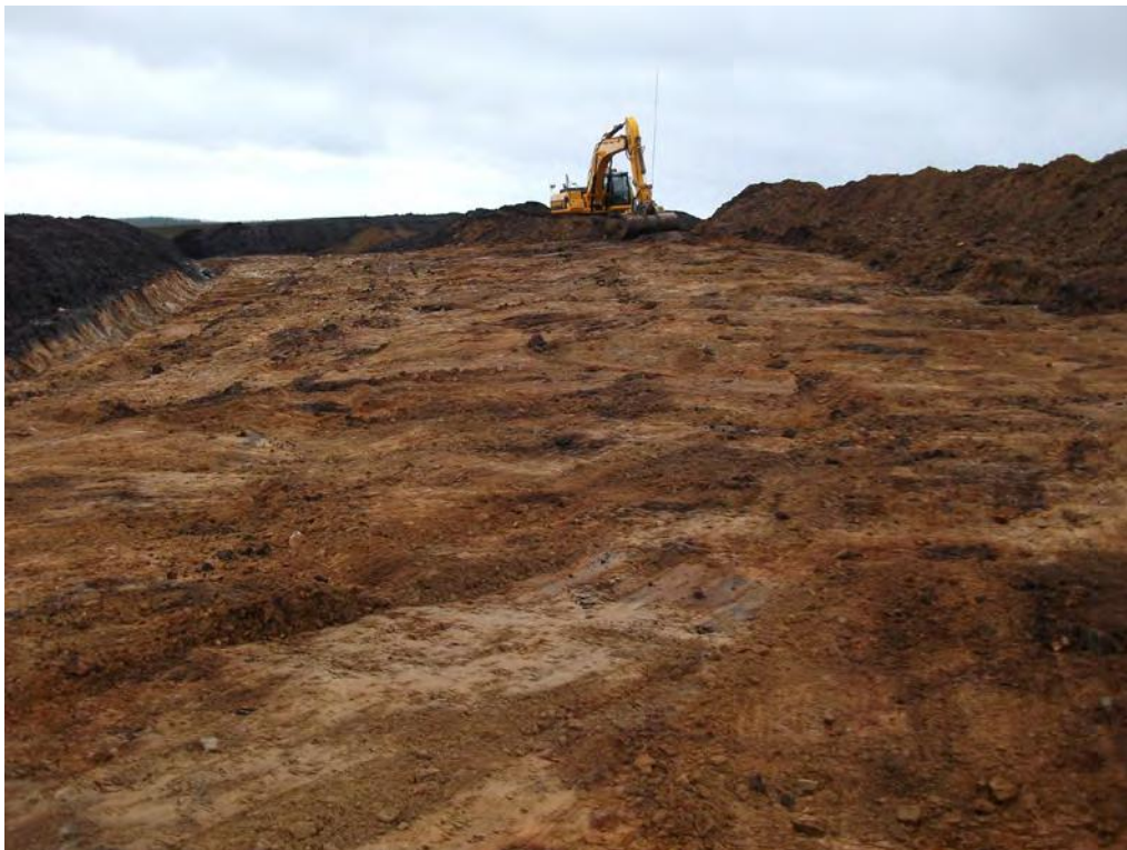
Fig. 8 Removing topsoil from Borrow Pit
