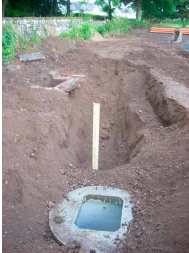
Fig. 2 - The route of the gravity sewer trench where it passes the top of the steps from the NE
