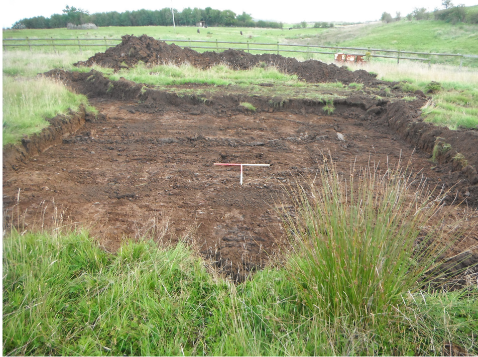
Fig. 2 - Turbine base stripped of topsoil from west
