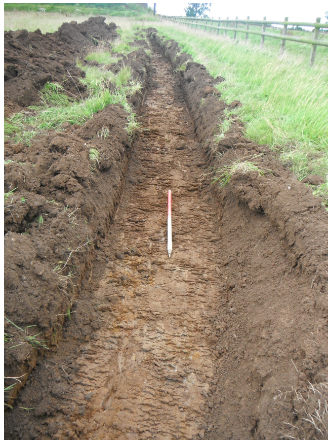
Fig. 3 - Topsoil stripping along cable trench
