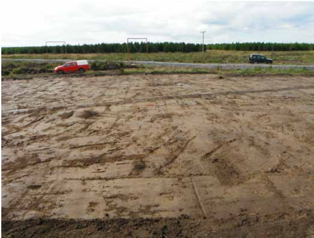
Fig. 5 - Turbine 3 stripped of topsoil, from north
