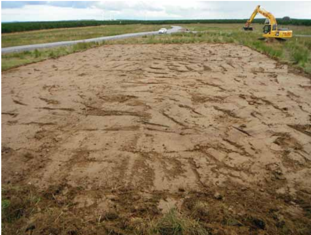
Fig. 7 - Turbine 4 stripped of topsoil, from north-west
