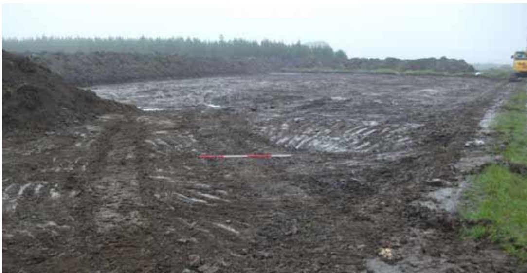
Fig. 3 - Compound area stripped of topsoil, from south
