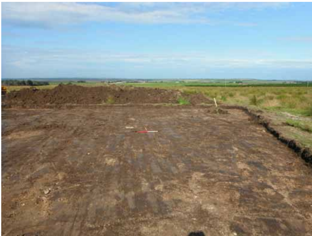
Fig. 8 - Electrical control building stripped of topsoil, from south
