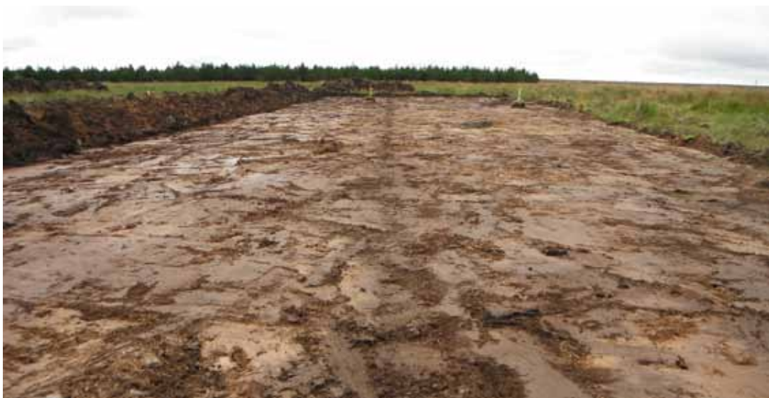
Fig. 4 - Turbine 1 stripped of topsoil, from north-west
