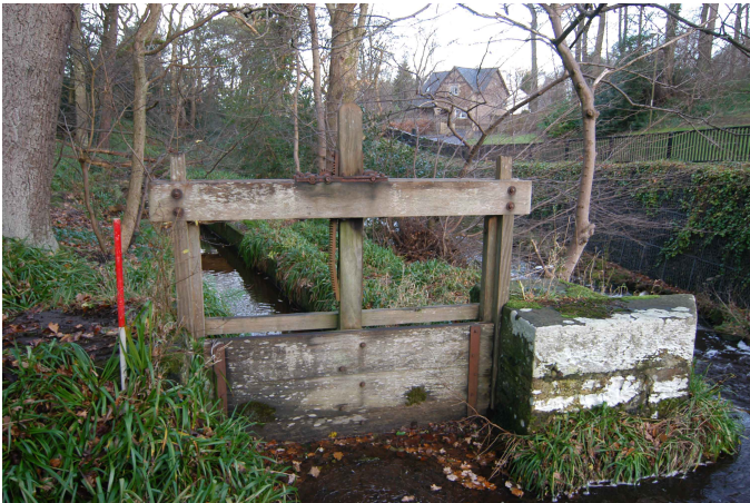
Figure 7: Detail of back of sluice
