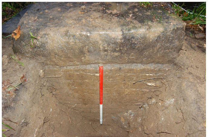
Figure 6: Section of test pit showing brick pier (005/1)
