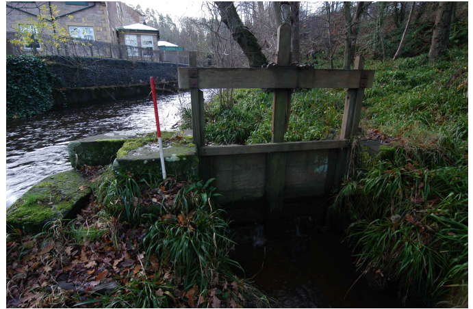
Figure 6: View of front of sluice
