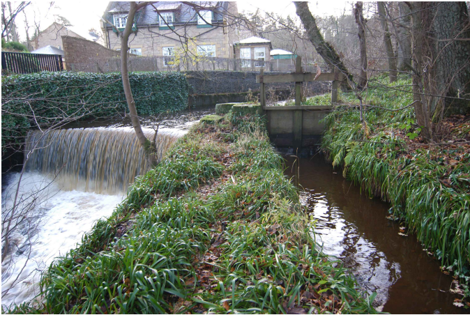
Figure 5: View of sluice within setting
