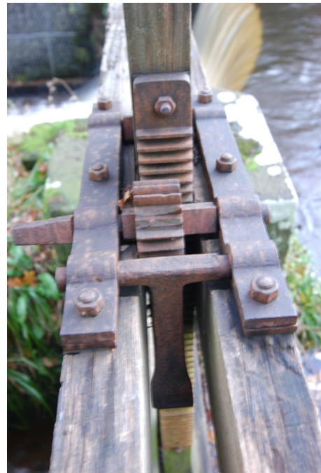
Figure 8: Detail of gate-winding mechanism
