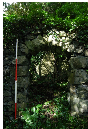
Plate 18: General view of the door surrounds and segmented arch
