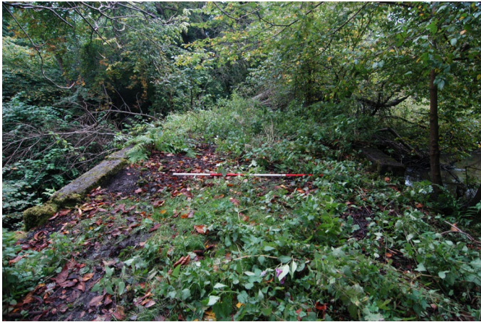
Plate 13: General view of the bridge deck looking south
