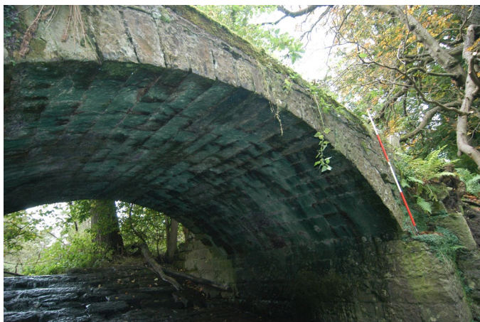
Plate 5: East-facing elevation, detail of the segmented arch voussoirs
