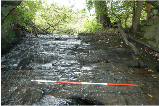
Plate 9: Overflow weir stonework on the west side of the bridge
