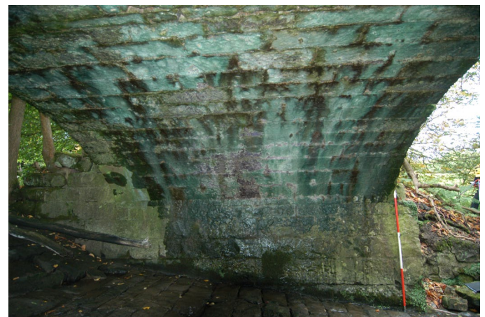
Plate 6: North abutment, south-facing ashlar stonework below the bridge and soffit stonework above
