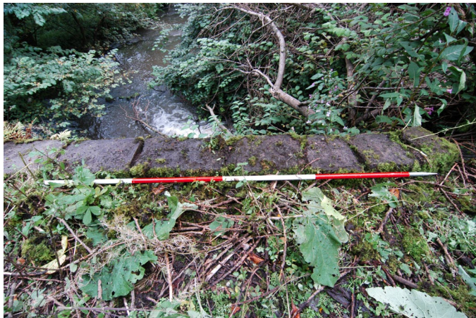
Plate 15: Kerb stones on top of the east-facing elevation, south end
