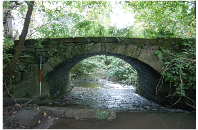
Plate 10: Mill Weir Bridge west-facing elevation
