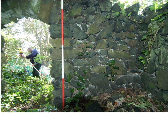
Plate 25: Interior wall fabric on the east side of the doorway
