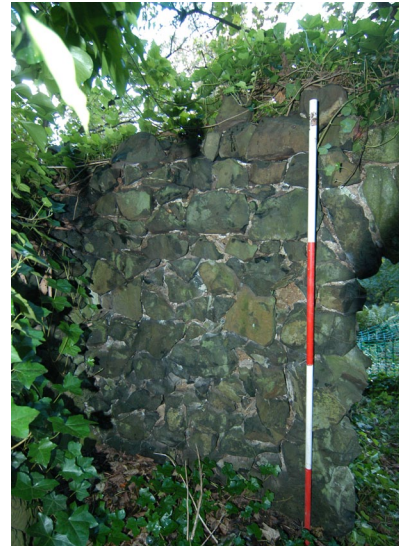
Plate 26: Interior wall fabric on the west side of the doorway
