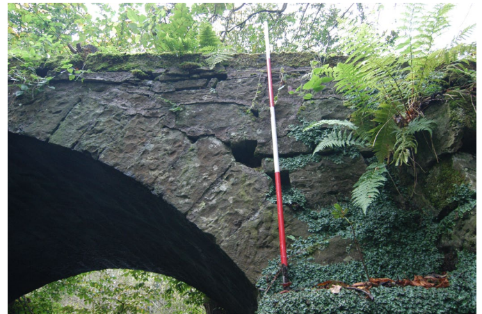
Plate 4: East-facing elevation, showing the spandrel above the arch
