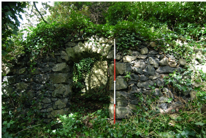
Plate 17: General Tam's Smokehouse south-facing elevation
