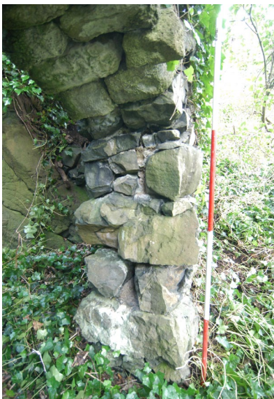
Plate 21: Wall core seen within the east side of the doorway
