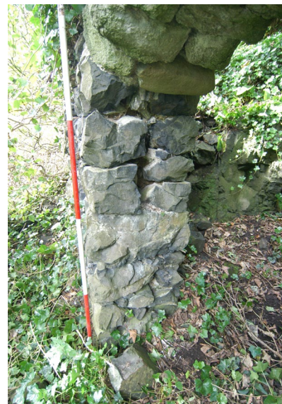
Plate 22: Wall core seen within the west side of the doorway
