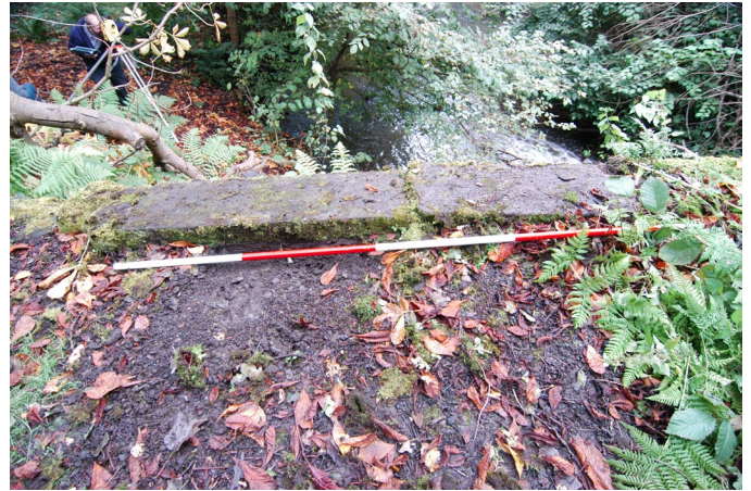
Plate 14: Kerb stones on top of the east-facing elevation, north end
