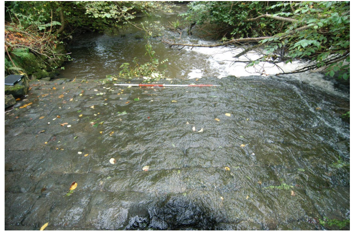
Plate 8: Overflow weir stonework on the east side of the bridge
