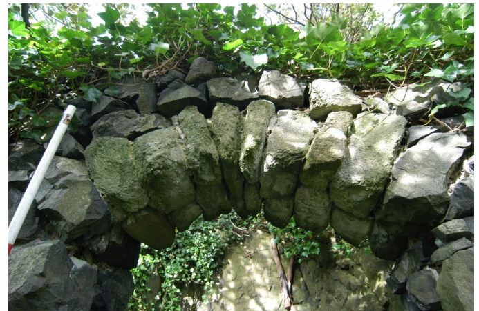
Plate 24: Close up of the interior segmented arch
