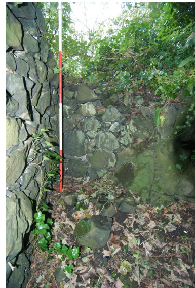
Plate 28: Infilling wall between the main interior elevation and natural rock (west side)
