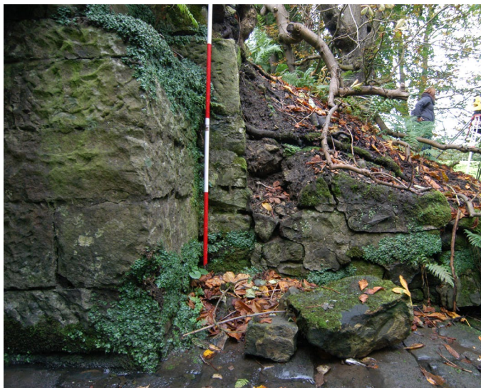
Plate 3: South-facing abutment showing erosion and stone displacement
