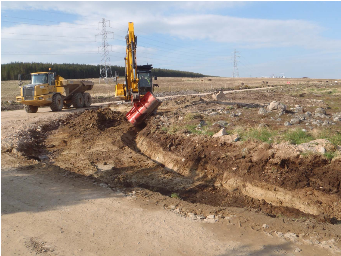
Fig. 4 Construction of Bell Mouth next to Cairn Field NJ04NW0017
