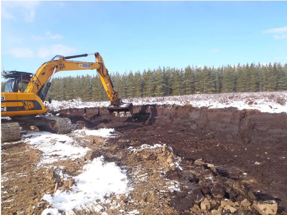
Fig. 7 Excavation of TP. 27 showing natural and depth of overlying peat
