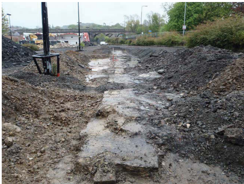
Fig. 5 Wall 005/007 from the north-west
