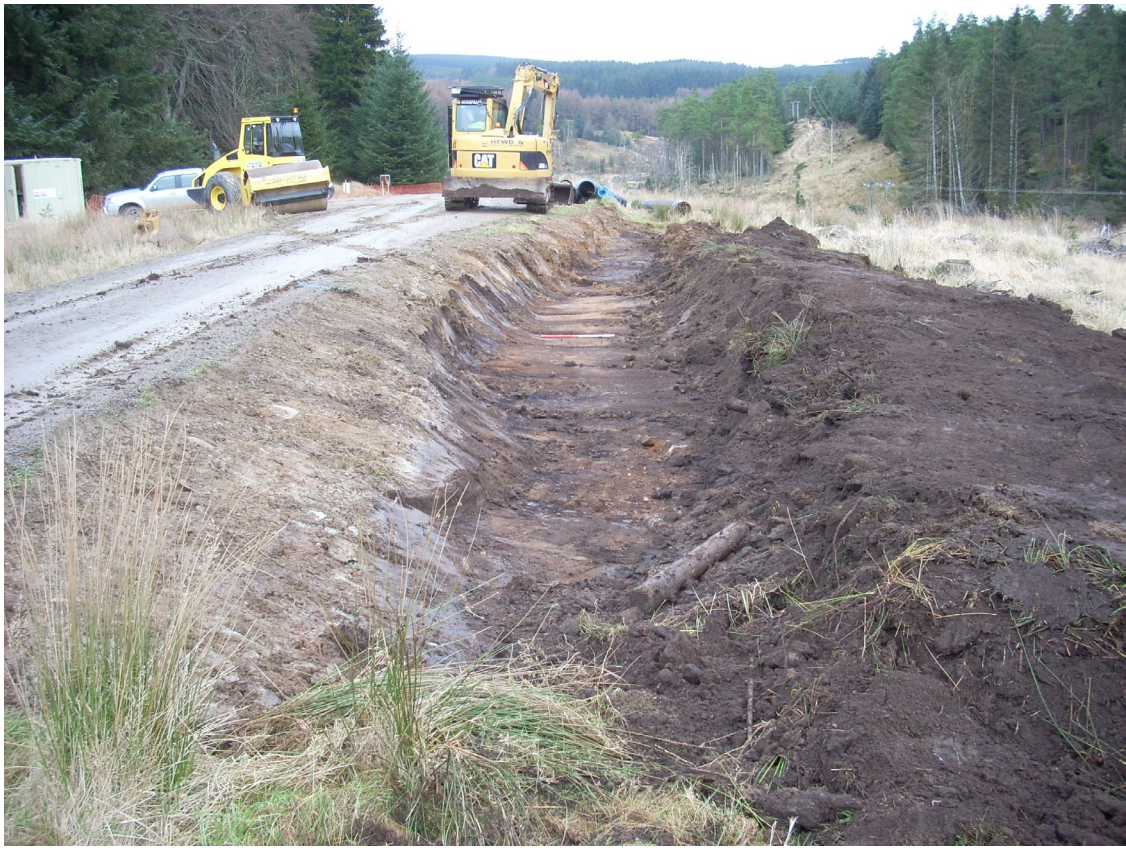
Fig 4: Road widening works for passing place
