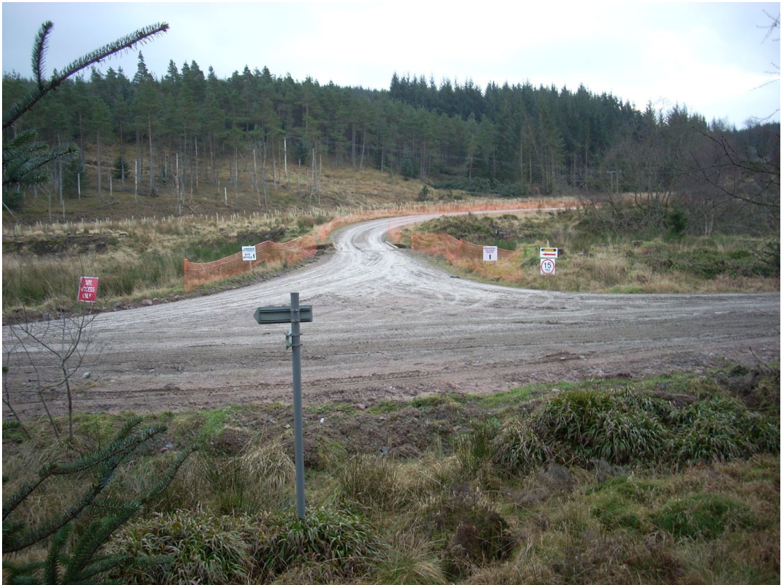
Fig 3: Scheduled area fenced, Site 1
