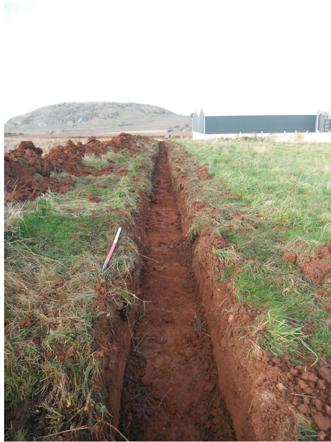
Fig. 6: Cable trench section looking north north west
