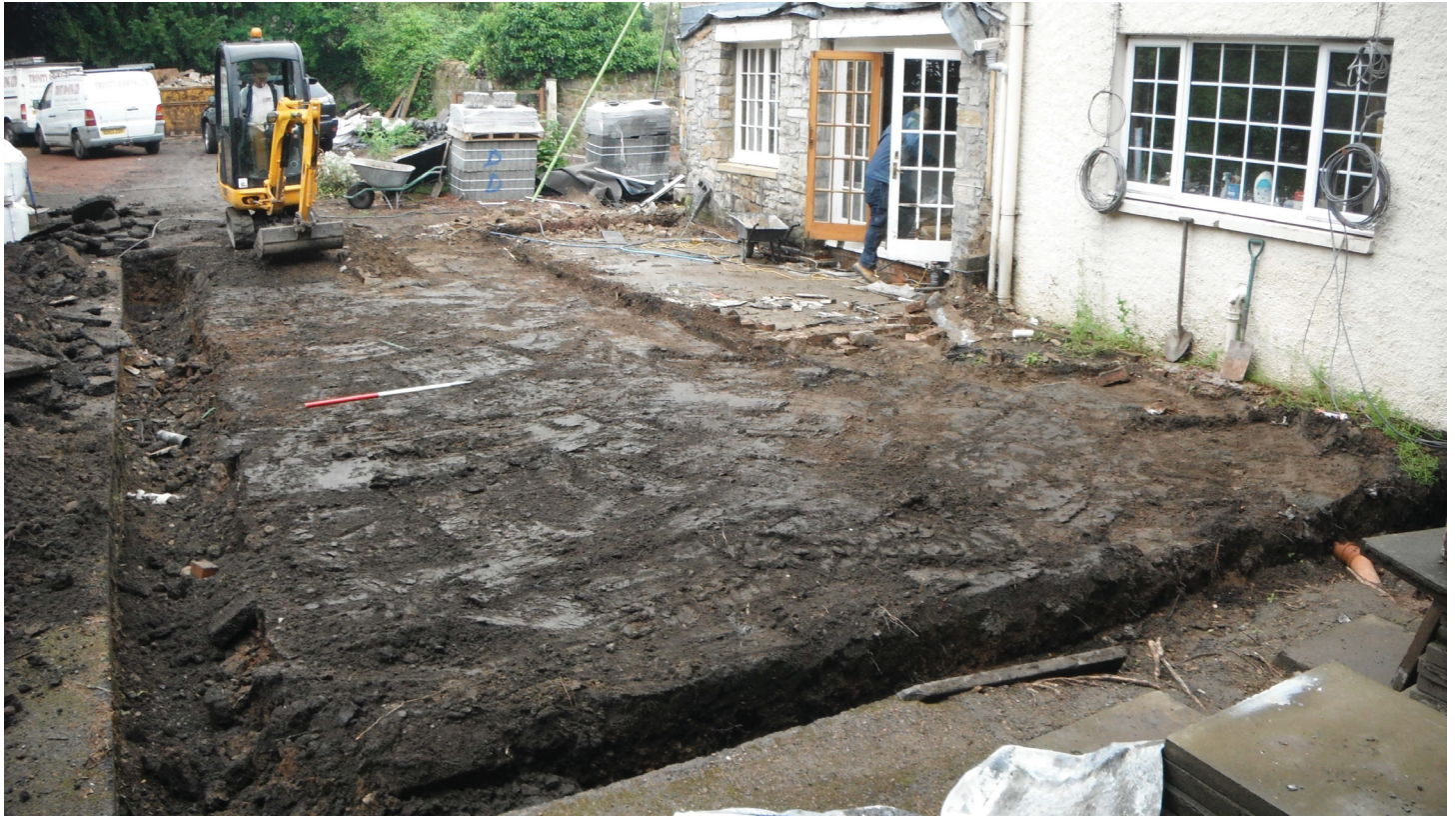
Fig. 3: Stripped area and foundations
