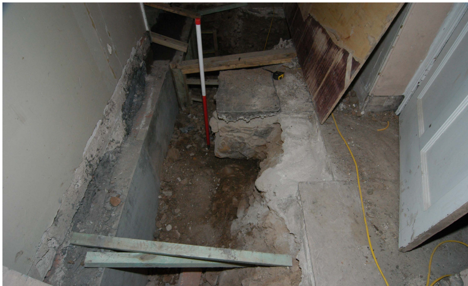
Plate 3: Basement corridor area B.48, exposed wall foundations recorded during underpinning work
