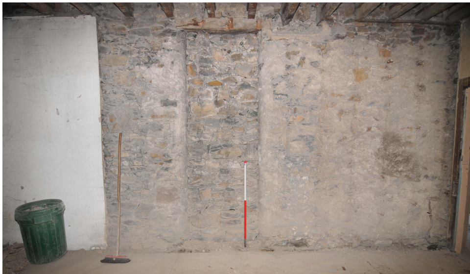
Plate 11: Storeroom B.28, general shot of the blocked opening on the south-west wall
