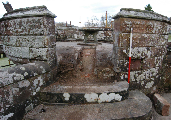
Plate 25: Game larder roof inspection trench within the domed interior of the parapet
