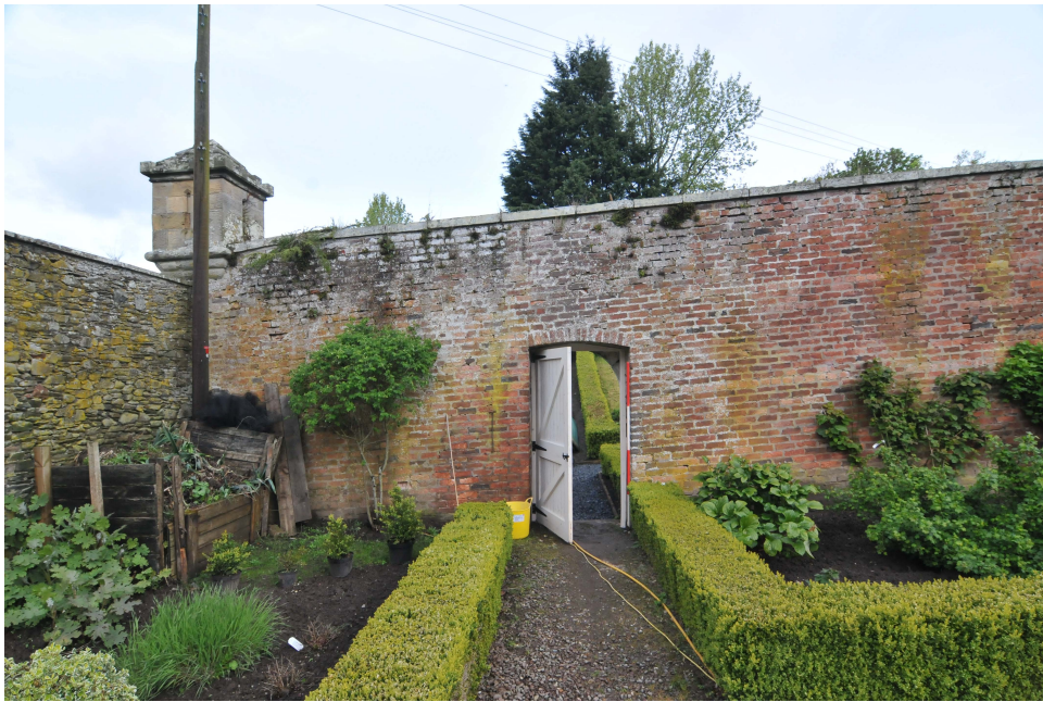
Plate 27: Kitchen garden wall entrance and wall detail
