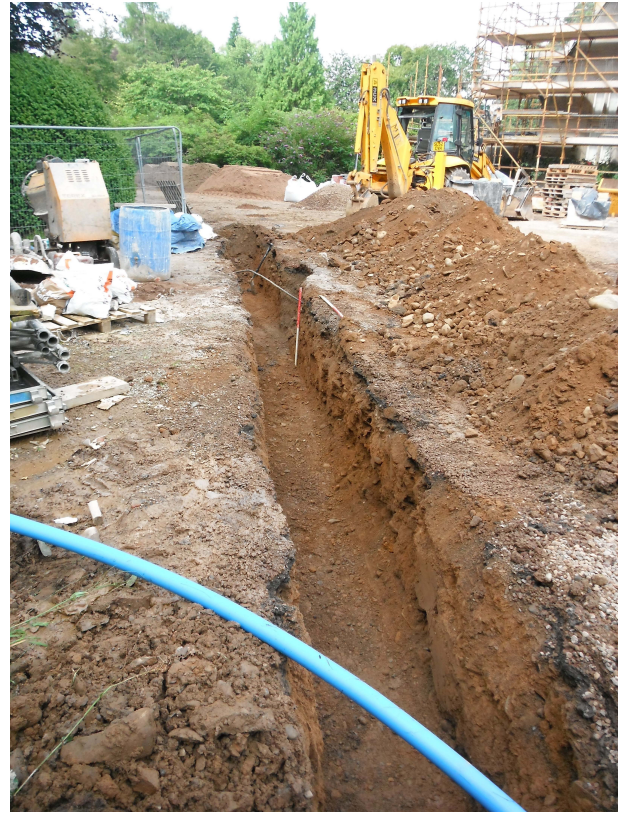
Plate 30: Water pipe trench leading to Abbotsford House
