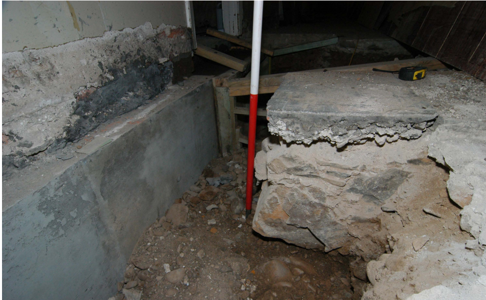
Plate 4: Basement corridor area B.48, close-up of exposed wall fabric
