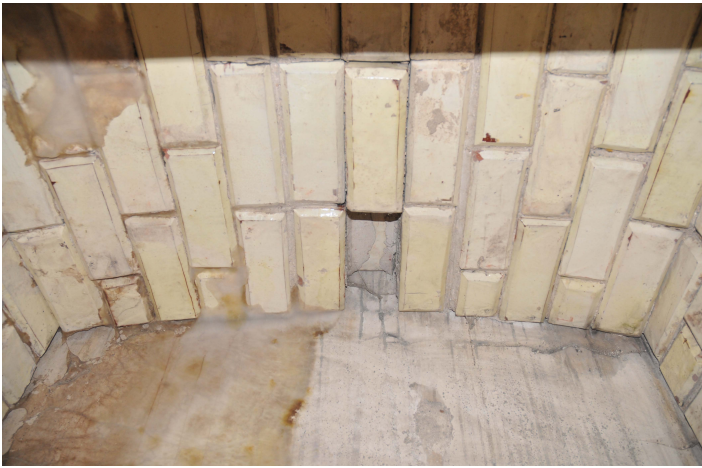
Plate 18: Room G.14 showing the arched brickwork on the cupboard interior
