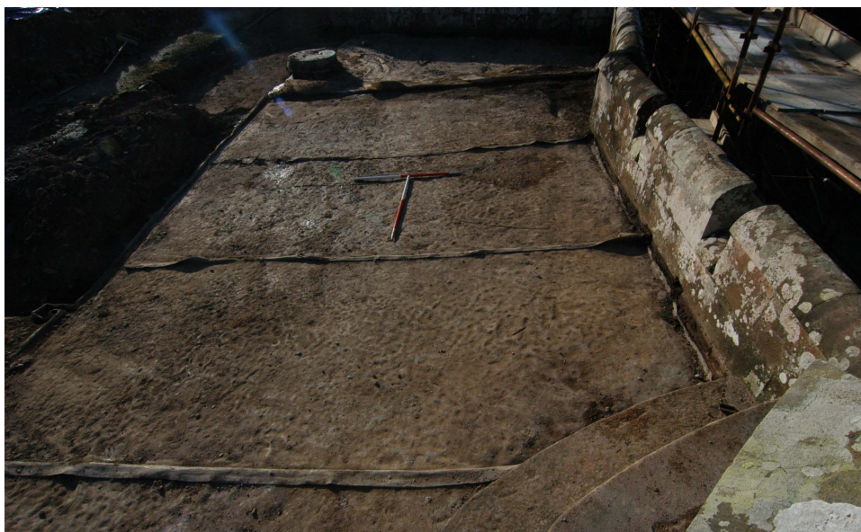
Plate 24: Lead sheets covering the roof of ice house and game larder
