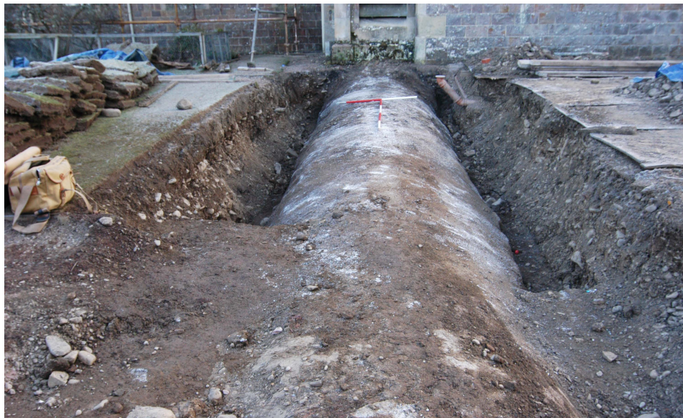
Plate 23: Ice house passage roof exposed prior to conservation work
