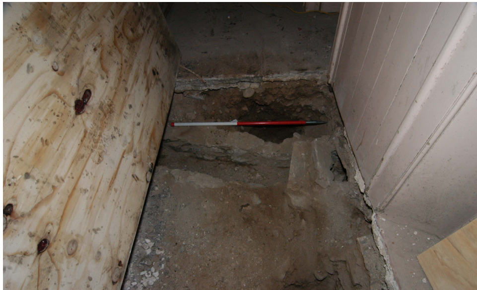
Plate 5: Basement corridor area B.17, general shot of exposed culvert
