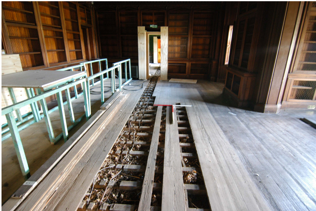
Plate 21: Library G.07 showing the exposed floor-joists exposed during refurbishment work
