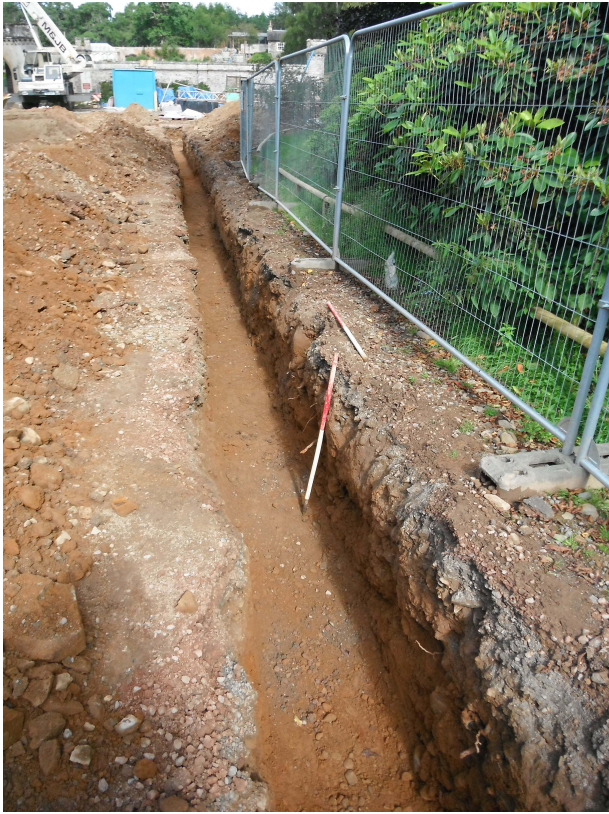
Plate 29: Water pipe trench leading to Abbotsford House
