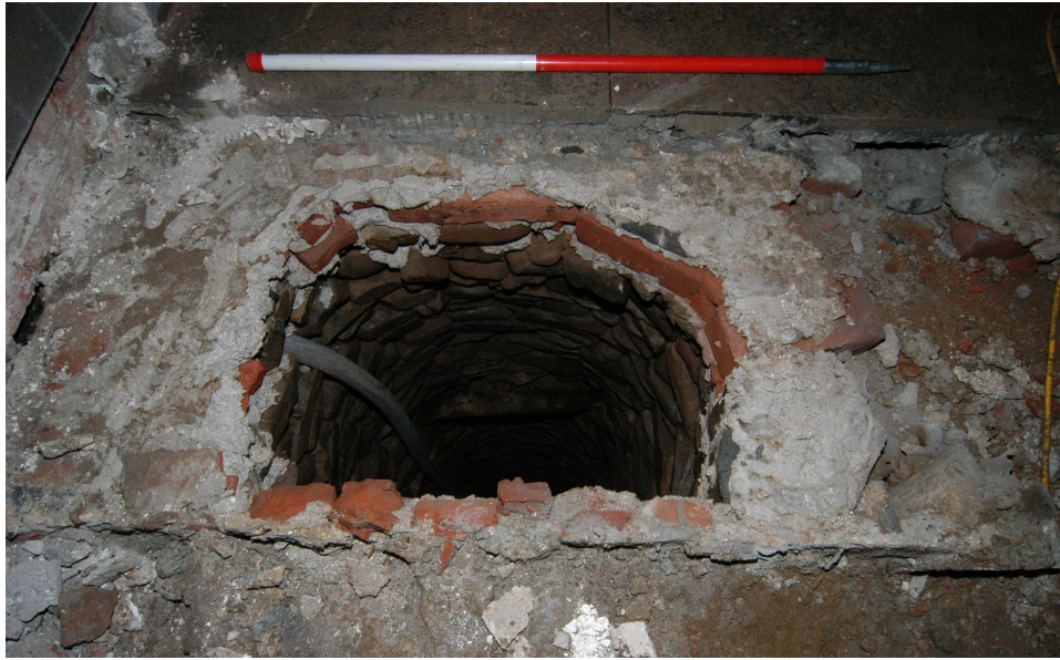
Plate 7: Hall B.38, exposed well with modern capping material
