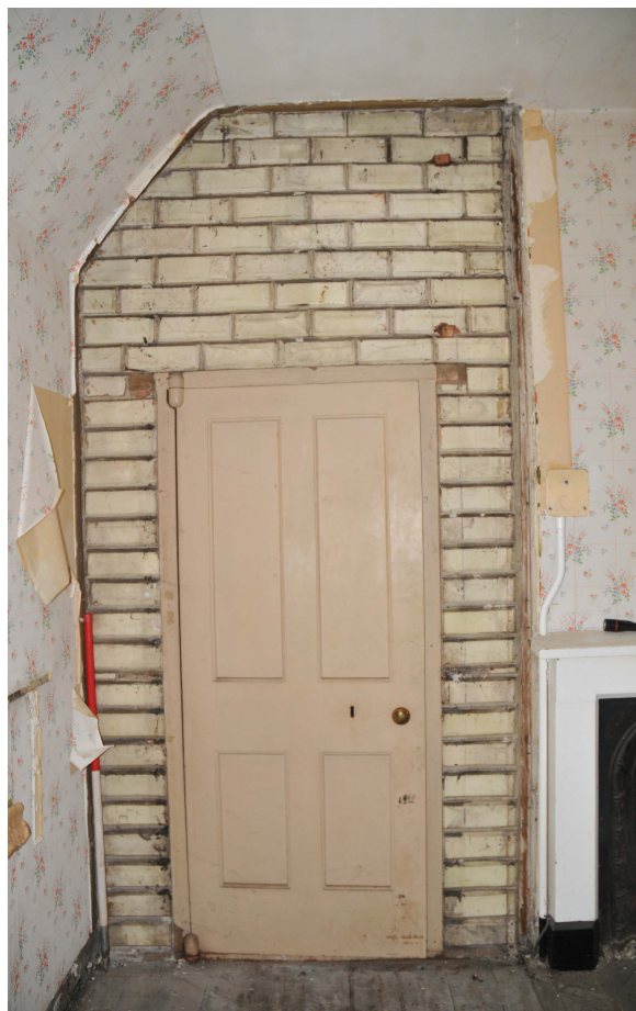
Plate 15: Room G.14 showing the cast-iron four paneled door
