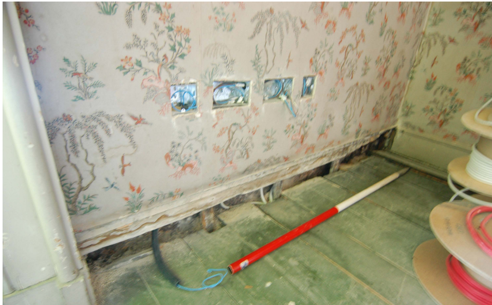
Plate 22: Room F.21, exposed cast-iron beam at the base of the wall
