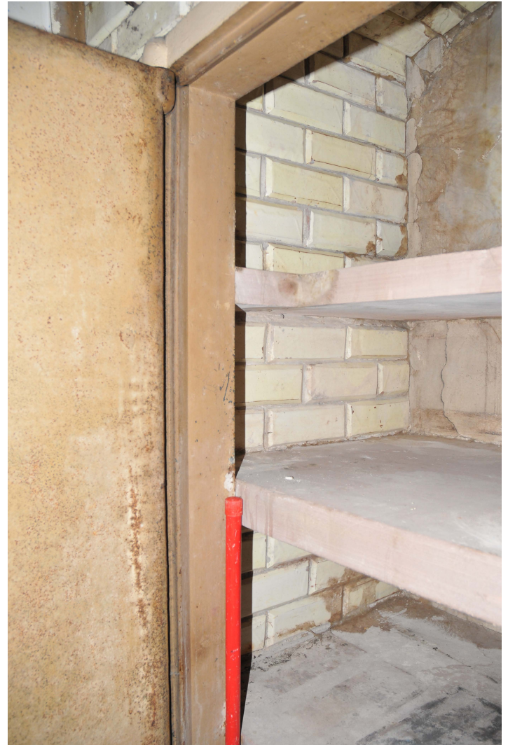
Plate 19: Room G.14 showing the arched brickwork
