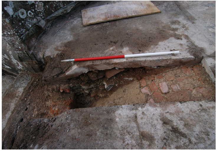
Plate 26: Game larder roof construction material exposed in section
