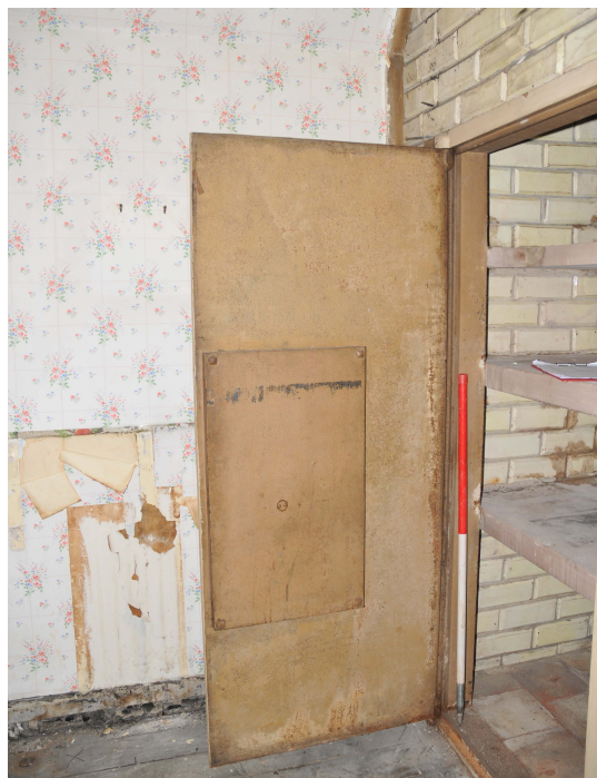
Plate 17: Room G.14 showing lock plate on the rear of the door
