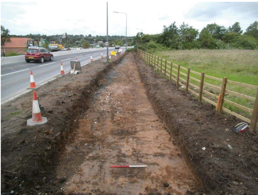
Plate 2: Area 4 following topsoil removal
