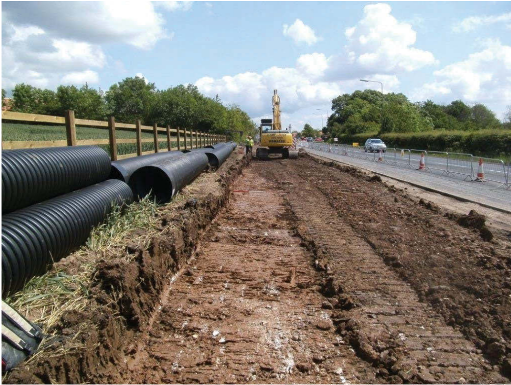
Plate 1: Area 1 during topsoil removal
