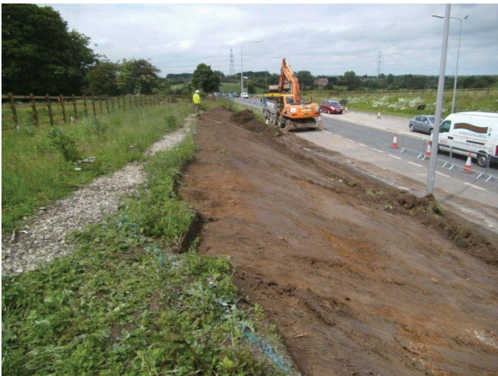
Plate 4: Area 9 following topsoil removal
