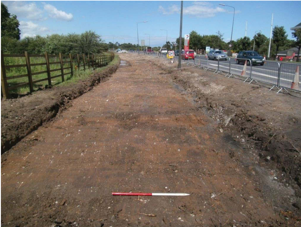
Plate 3: Area 5 following topsoil removal
